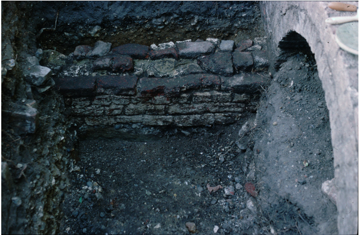
Figure 87. The northern channel wall at the culvert exit [CU17]. South side.
