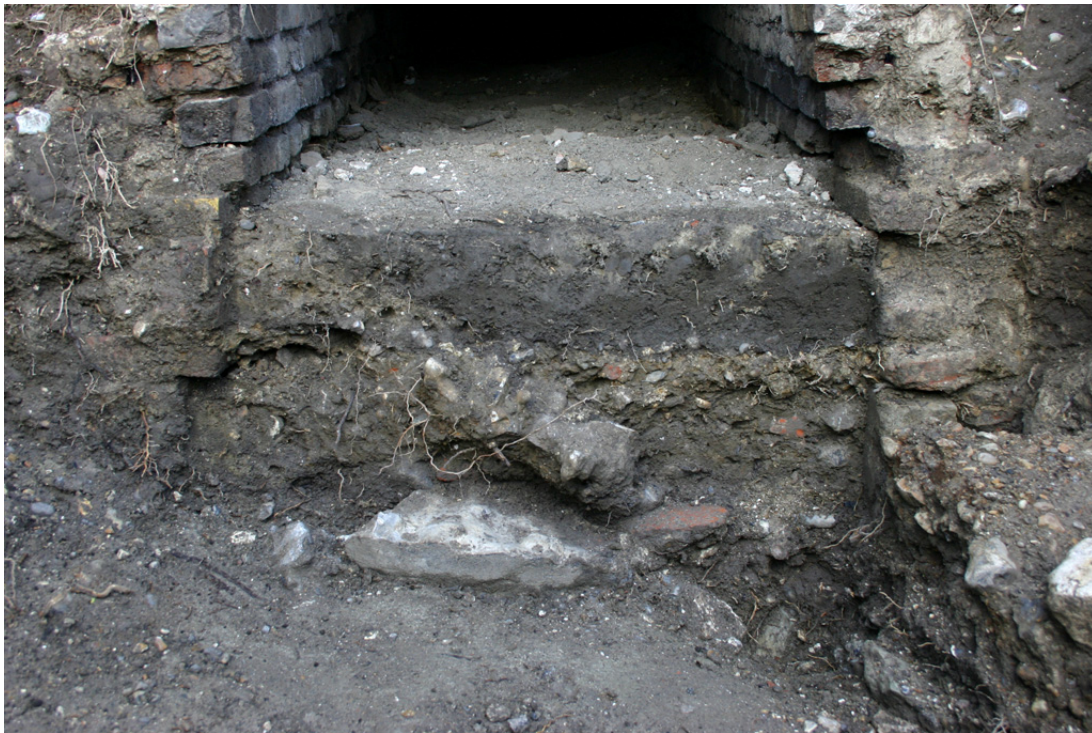
Figure 84. The west end of culvert section 3.
