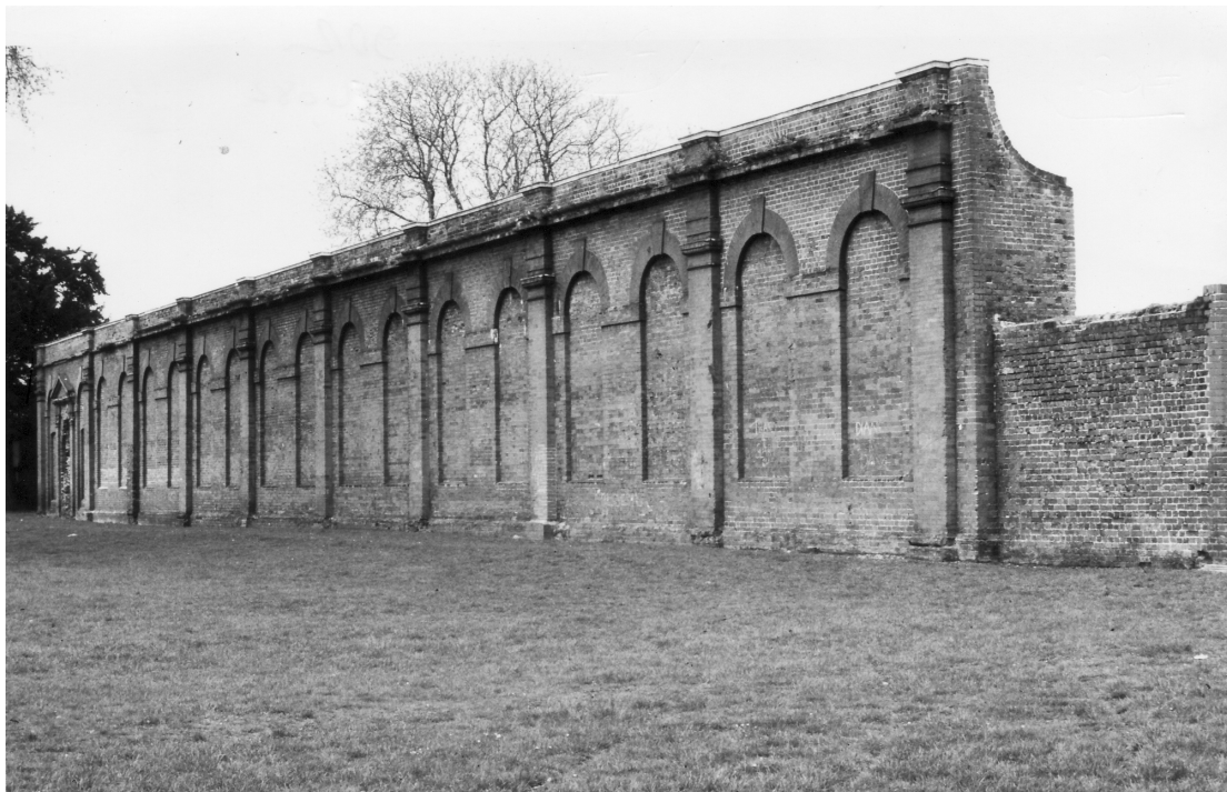
Figure 36. The north side of the Orangery wall from the west end.
