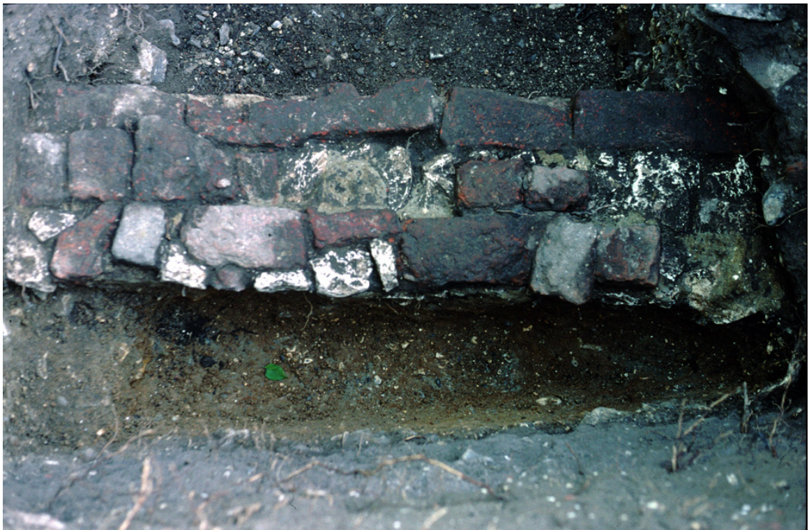
Figure 88. The northern channel wall at the culvert exit [CU17] from above.
