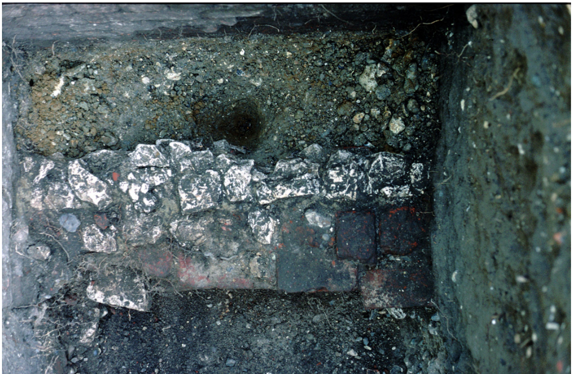
Figure 86. The southern channel wall at the culvert exit [CU15] from above.
