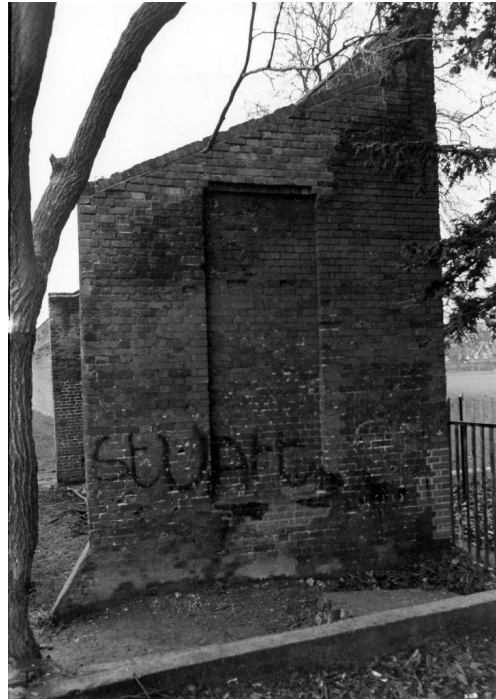
Figure 44. The east end of the wall.
