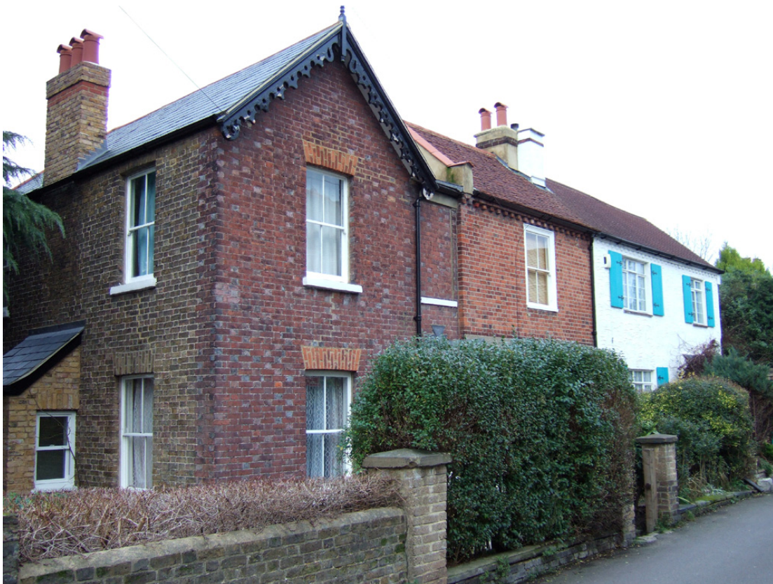
Figure 64. 12 and 14 Church Lane. The two cottages in the background may be of early eighteenth century date. The section in the foreground is clearly a Victorian addition.
