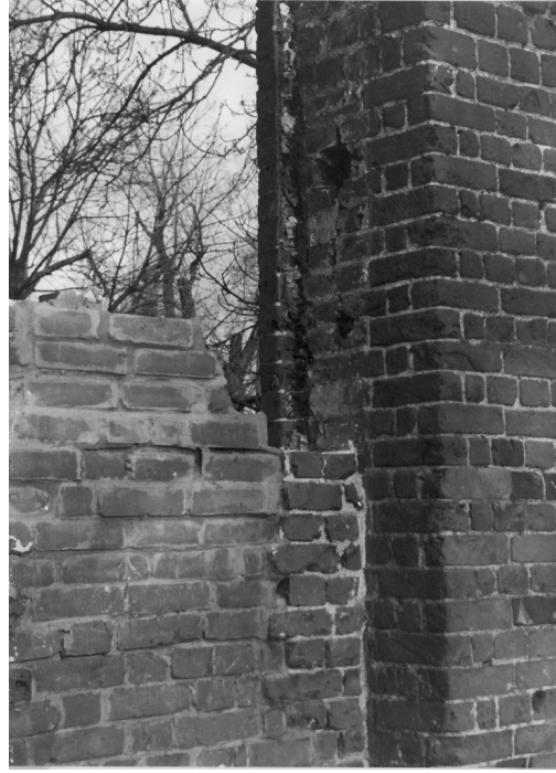
Figure 47. East side of the western window.
