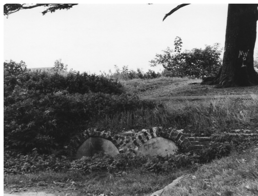
Figure 31. The cascade culverts in 1987.
