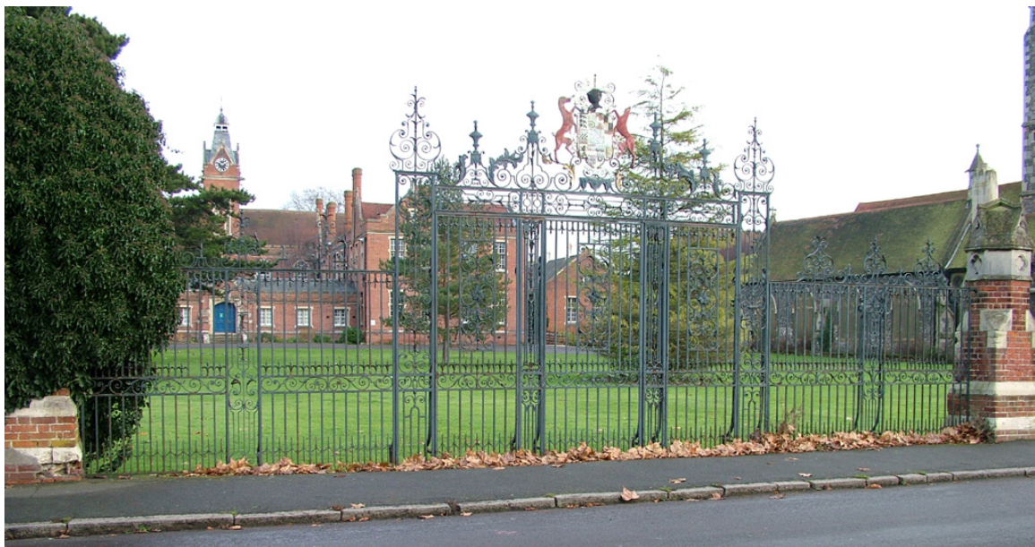
Figure 103: The west gates in January 2006.
