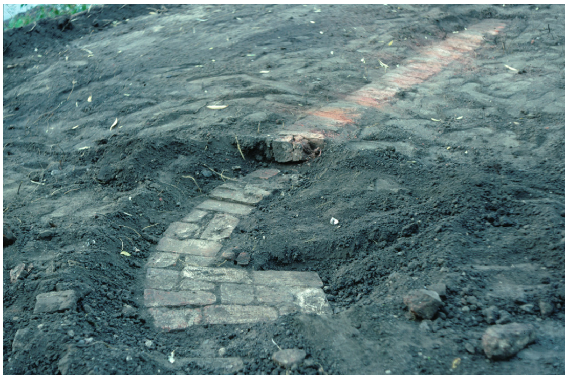
Figure 99. Foundation of a retaining wall on the east side of the channel at the exit from the east lake. Looking north-west during the flood alleviation work in 1990-1.
