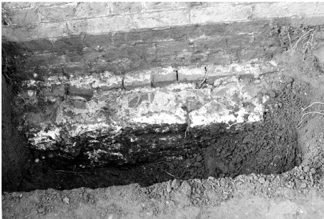
Figure 61. The foundation [CT29] on the south side of the Orangery wall.
