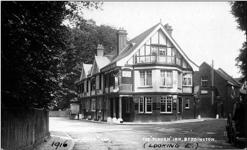
Rebuilt in 1897-98, the pub as seen in 1916 with the main entrance to the yard beneath the 'Livery & Bait Stables' arched sign that linked the pub to the stable block.
