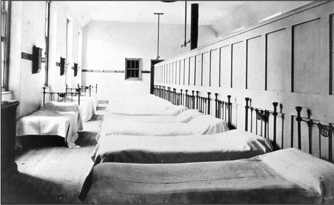
One of the Orphanage dormitories.
