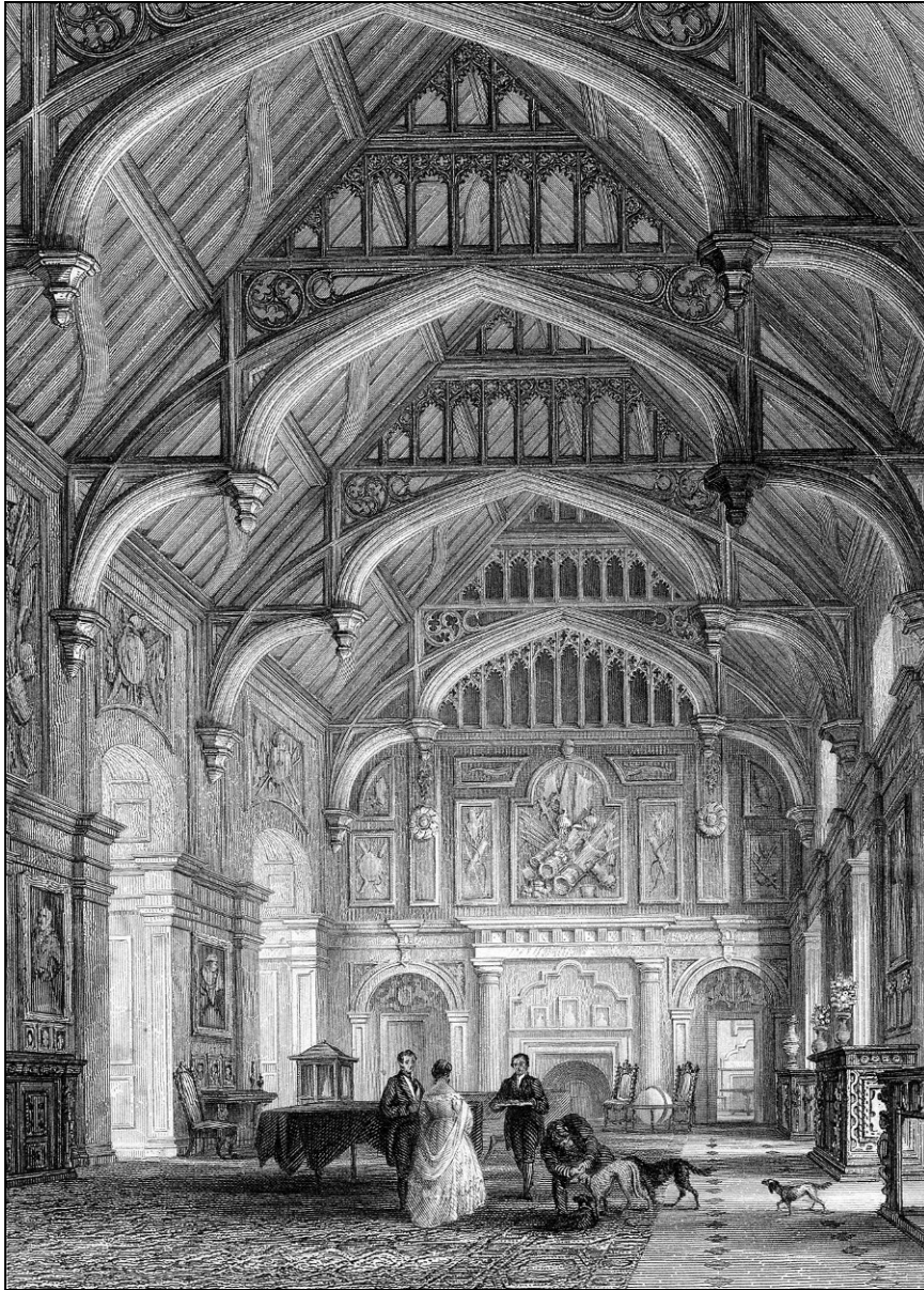
The magnificent hammer-beam roof within the great hall as depicted in 1850. Of late 15 th or early 16 th century dating it is a survivor of at least two, possibly three older houses.
