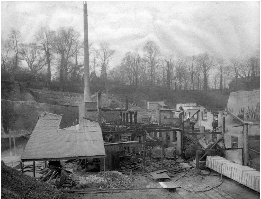
Messrs Jesse Clack & Sons brickworks after the fire in April 1908. The works stood enclosed within a deep sand excavation, now site of Sherwood Park School. Croydon Road lies behind the wooden fence in the background while high on the skyline to the right amid the trees stands 'The Banks'.
