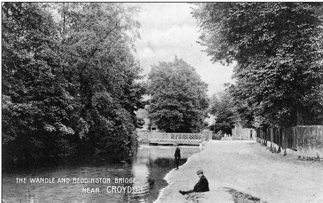
Completed in September 1893, an iron girder bridge replaced the footbridge. A ford to give horse drawn vehicles access via the river to the mill upstream, was retained.
