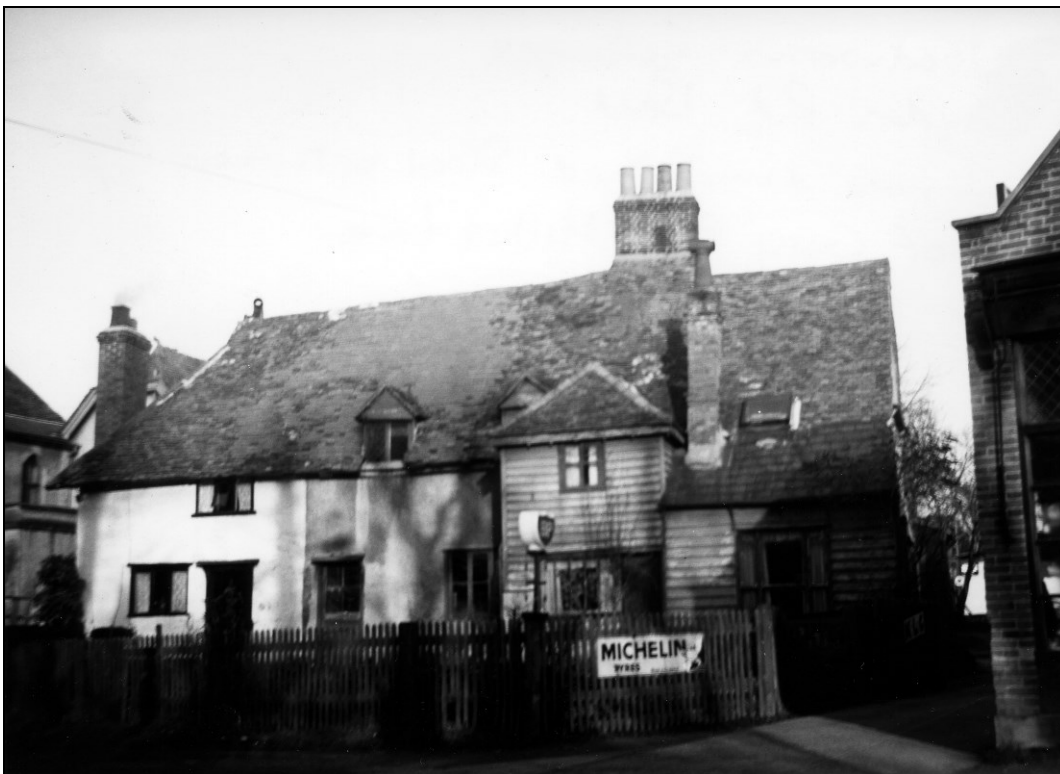
'Wormwood' or 'Sandy Hill Cottages' stood between Guy Road and Hilliers Lane before being demolished in 1960.
