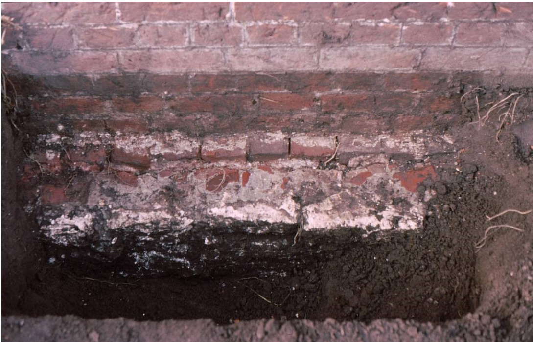
Figure 51. The top of foundation [CT29] next to the orangery wall.
