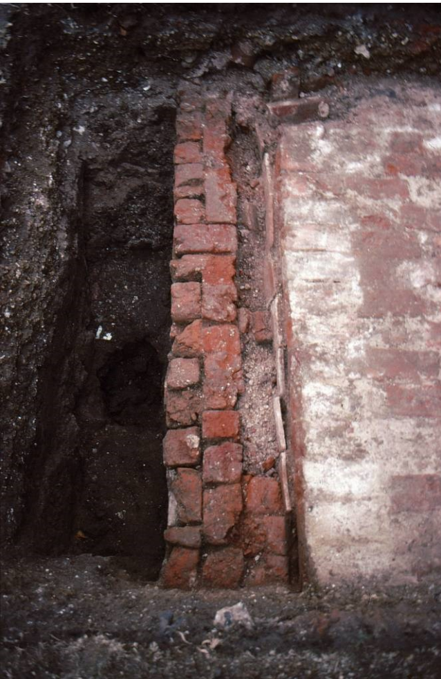
Figure 48. A section of foundation [CT22] has been removed to expose the peg tiles fixed to the south face of foundation [CT21].
