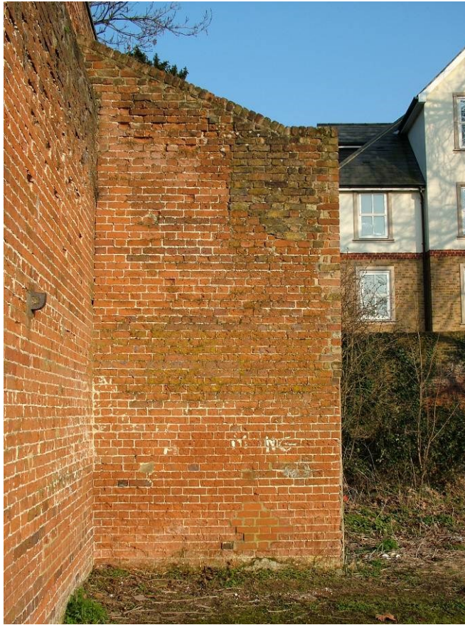
Figure 20. The west side of the west wall of the lean-to.
