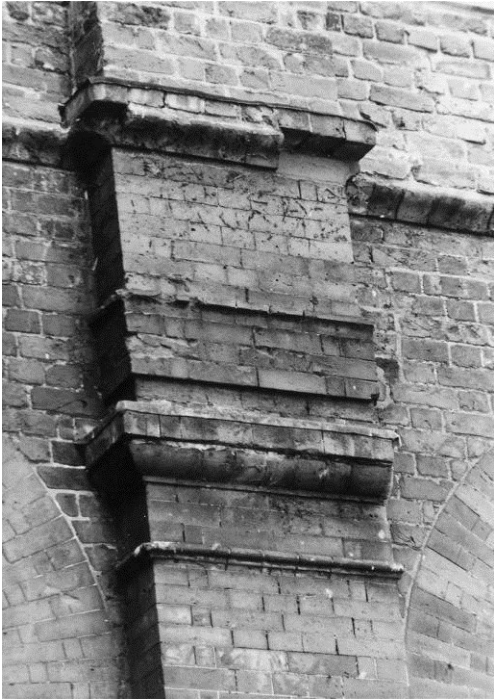
Figure 12. The top of pilaster 2.
