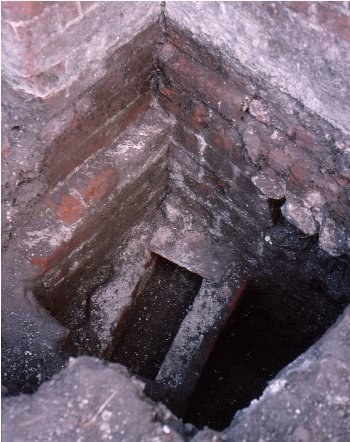
Figure 27. Trench CR with the drain. The end of the orangery wall on the left; the stub wall to the right.
