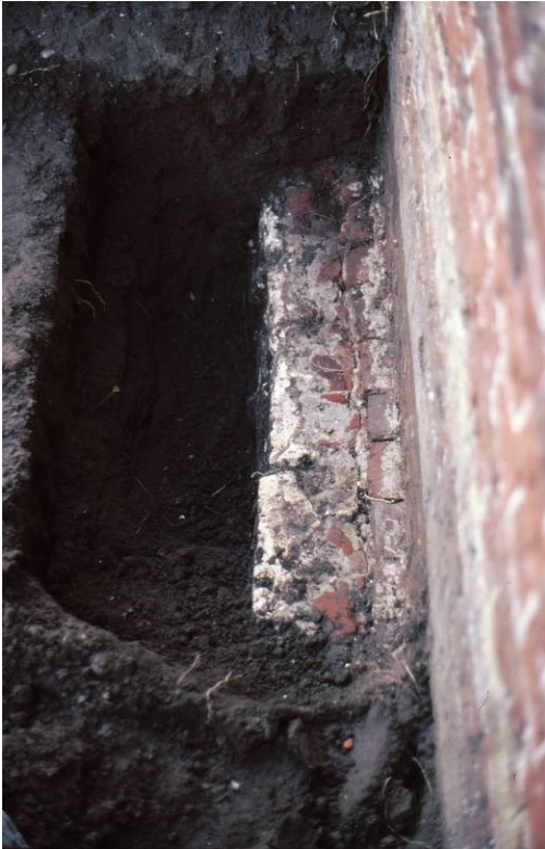
Figure 52. Foundation [CT29] looking west with the orangery wall on the right.
