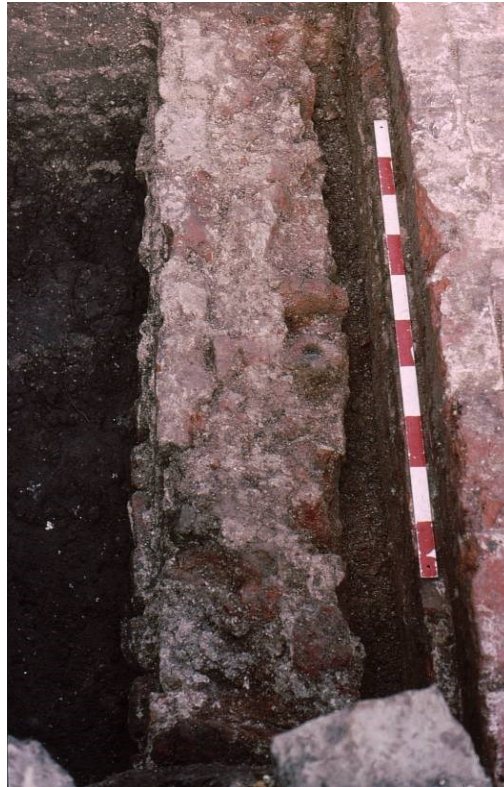
Figure 3. Foundation [CT30] with [CT21] to the right.
