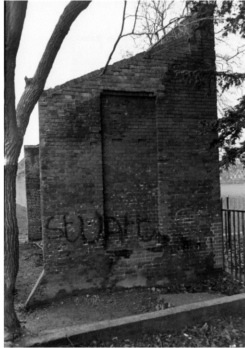
Figure 13. The east end of the wall.
