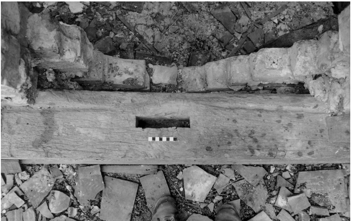
Figure 83. The centre of north truss in cottage 1B. Seen from above showing the mortise for a crown post or king post. Scale 8cm. 30 August 1982.
