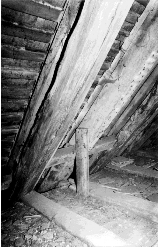
Figure 10. Cut rafter 10 with a little 'purlin' on the west side of cottage 1. Collars at the bottom of the photo.
