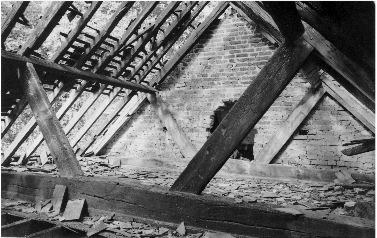
Figure 82. Roof of 1B. NW corner on the left. 29 August 1982.
