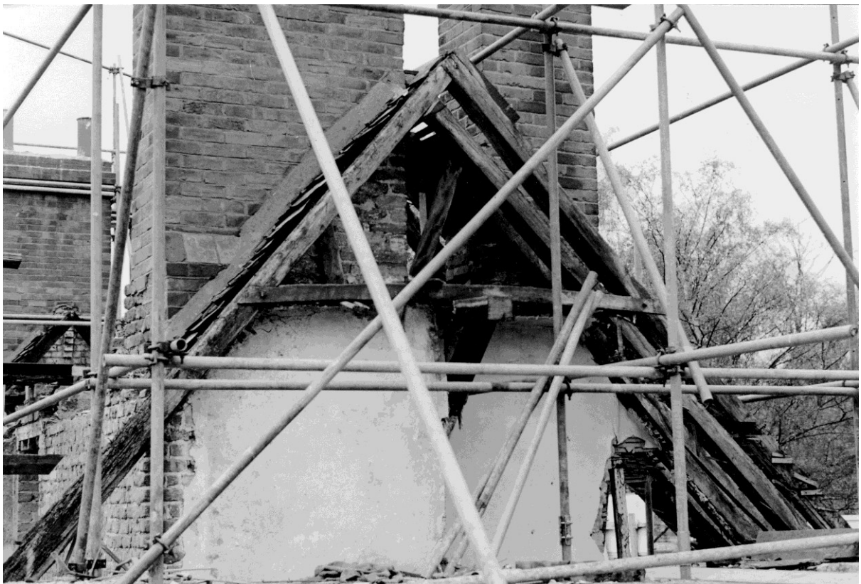
Figure 38. The east and west chimney-stacks (left and right) during conversion work.
