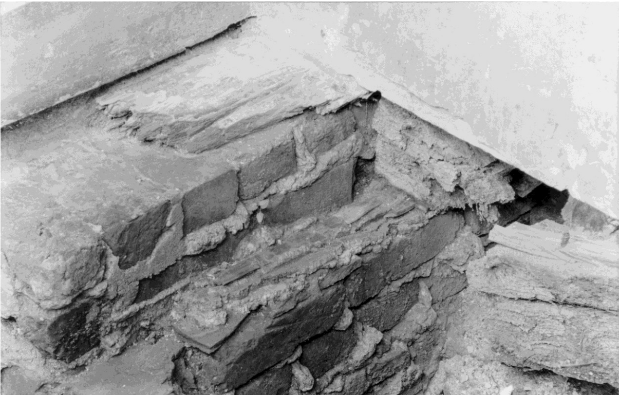
Figure 47. Detailed view of the two ledges shown in figure 46.
