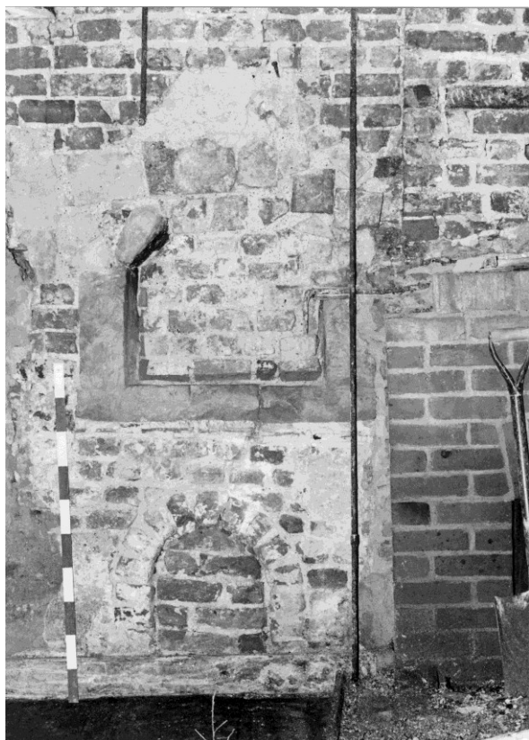
Figure 51. The blocked door and ash pit for the earliest oven in the south wall of room 1-5.
