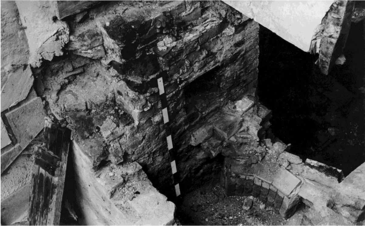
Figure 58. The east side of the east chimney-stack by the ovens. Note the unblocked flue to the right of the scale.
