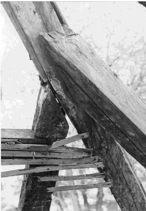
Figure 6. The hip on the north end of the cottages in 1986-7. Note the gap for a dormer window on the left and the cut rafter to the right of it, perhaps the site of an earlier dormer.
