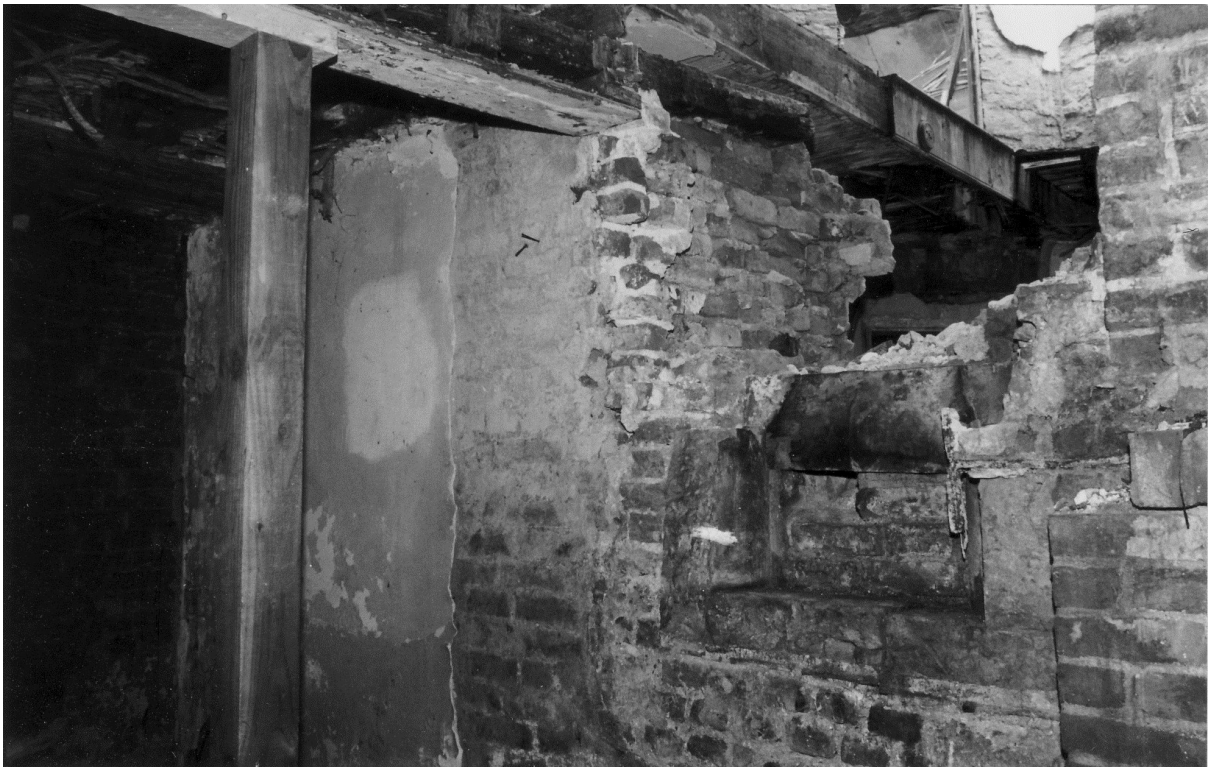
Figure 53. The oven and the south wall of room 1-5 looking south east.
