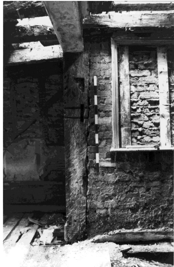
Figure 18. The bottom of post 2E showing a surviving section of ground sill resting on a brick foundation.
