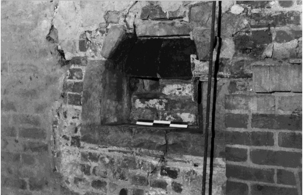
Figure 52. The door of the earliest oven with the blocking partly removed.
