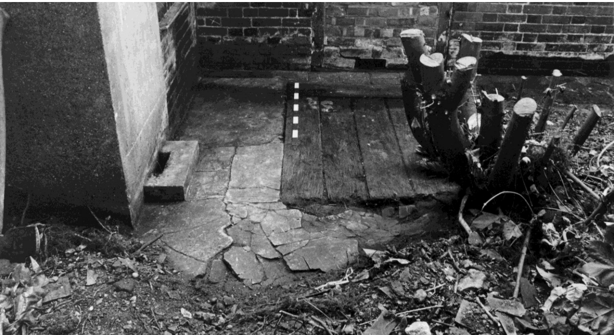
Figure 34. The corner between the extension of room 1-5 (left) and east wall of room 1-4 (right) showing the floor of the structure built against room 1-4. Blocked door to room 1-4 in the background.
