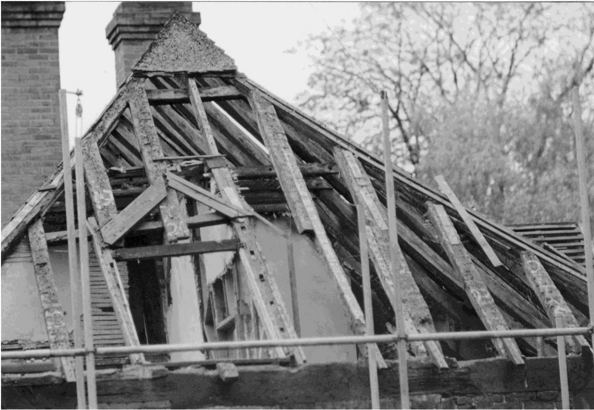
Figure 6. The hip on the north end of the cottages in 1986-7. Note the gap for a dormer window on the left and the cut rafter to the right of it, perhaps the site of an earlier dormer.
