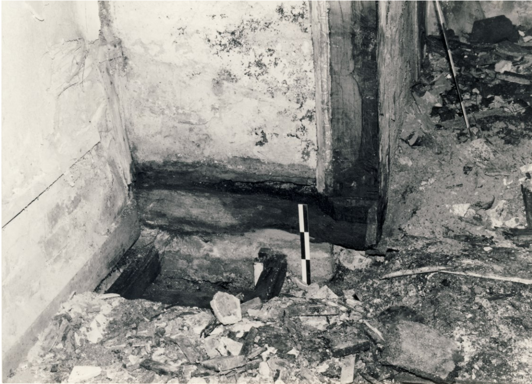
Figure 18. The bottom of post 2E showing a surviving section of ground sill resting on a brick foundation.
