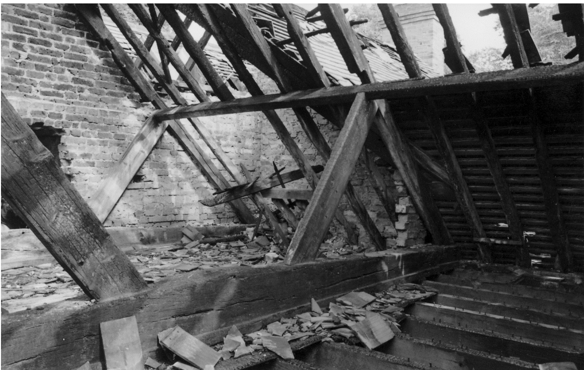
Figure 81. Roof of 1B looking NE. 29 August 1982.
