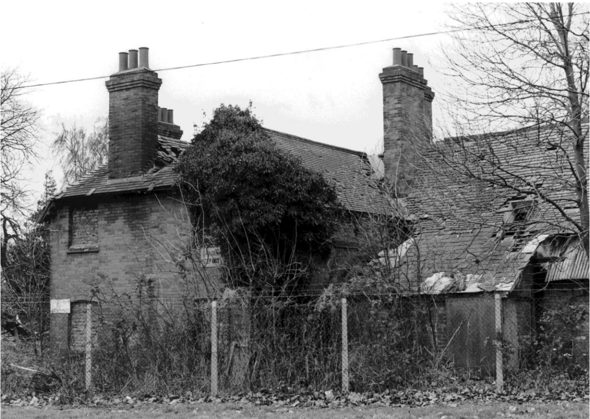
Figure 79. The extension to the rear of cottage 1A with cottage 1 to the right.
