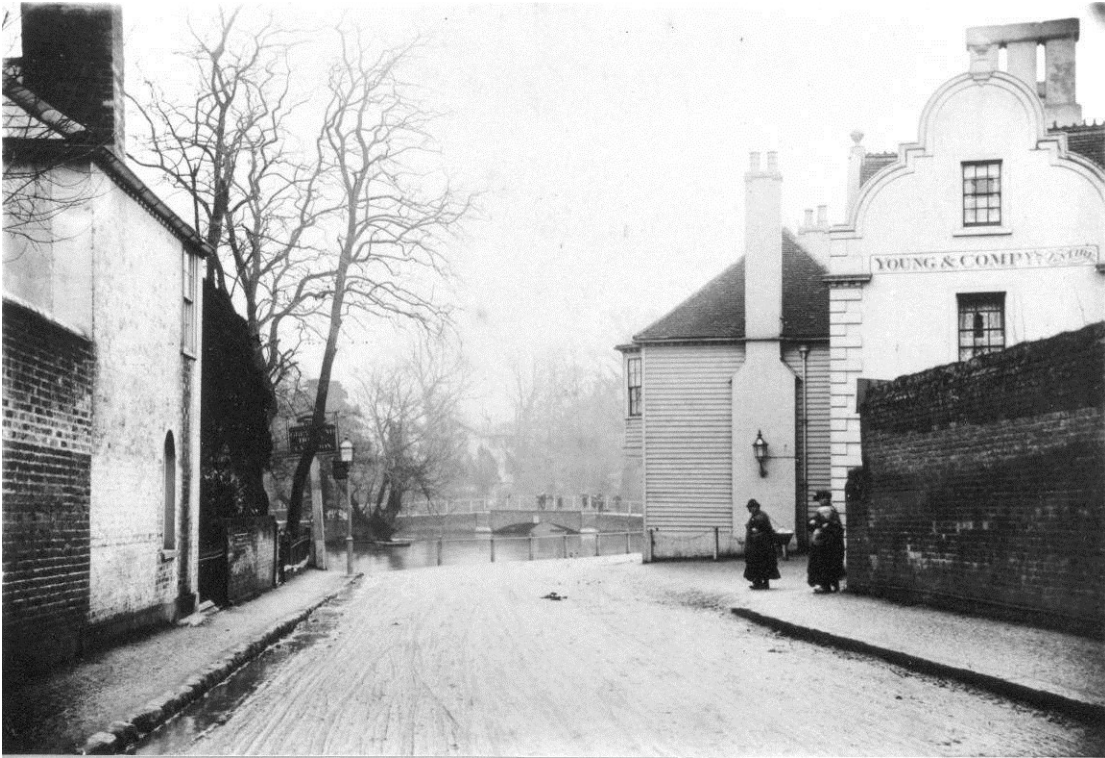
Figure 7. The Pound Street building or back extension to Honeywood. Note the water running down the gutter. Is this ground water seepage or rain?
