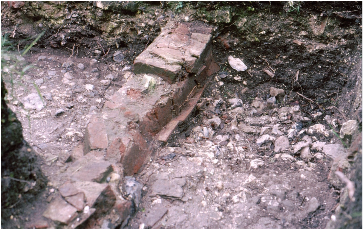
Figure 39. The southern end of the East Area looking east showing the damaged foundation [HD13].
