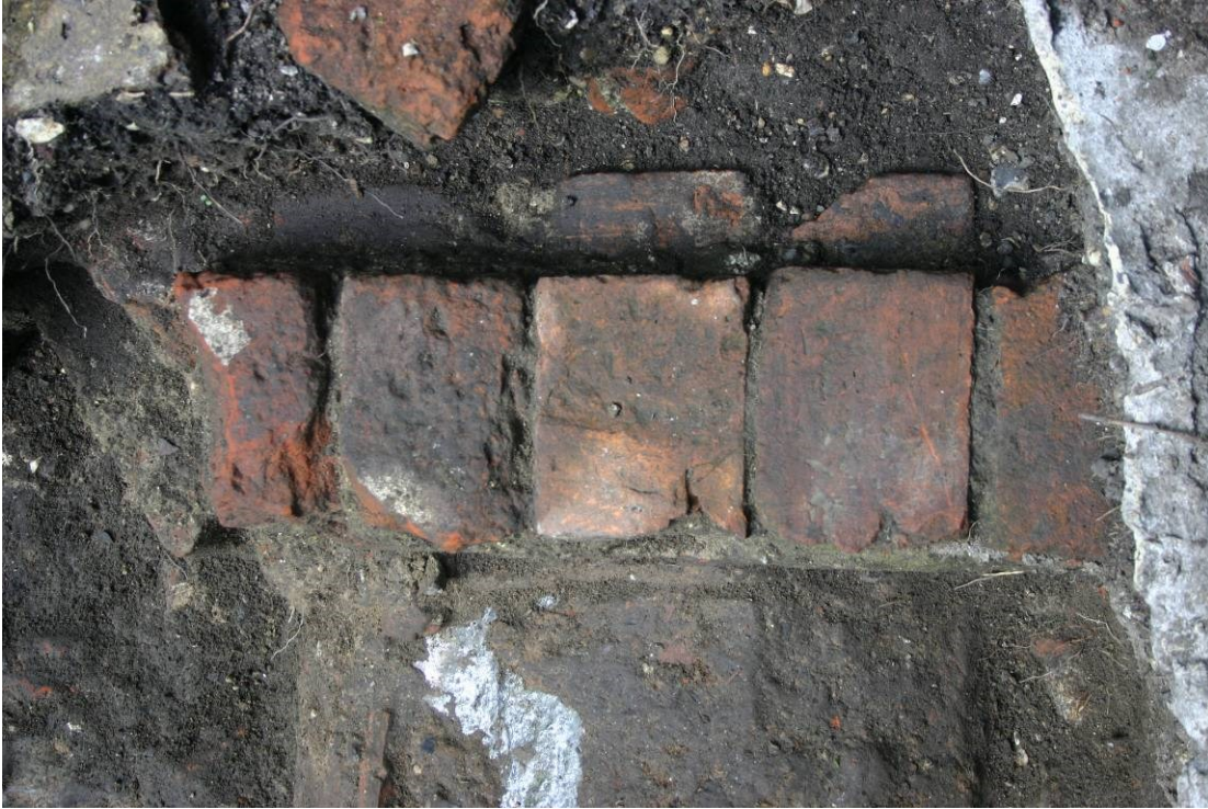
Figure 58. The top of retaining wall [C7]. North at the top.
