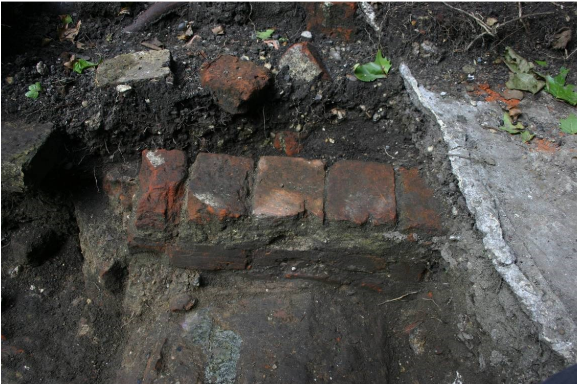
Figure 59. The south side of retaining wall [C7].
