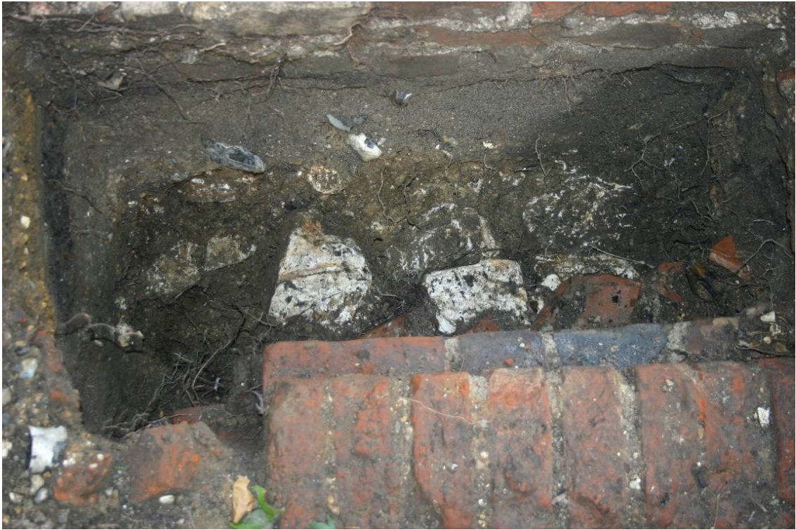
Figure 46. The chalk foundation of wall [B14]. East at the top.
