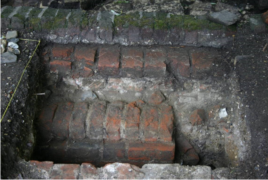
Figure 44. From top to bottom: the existing pond retaining wall in dark brick, the inner pond retaining wall [B3] and wall [B14]. Looking west.
