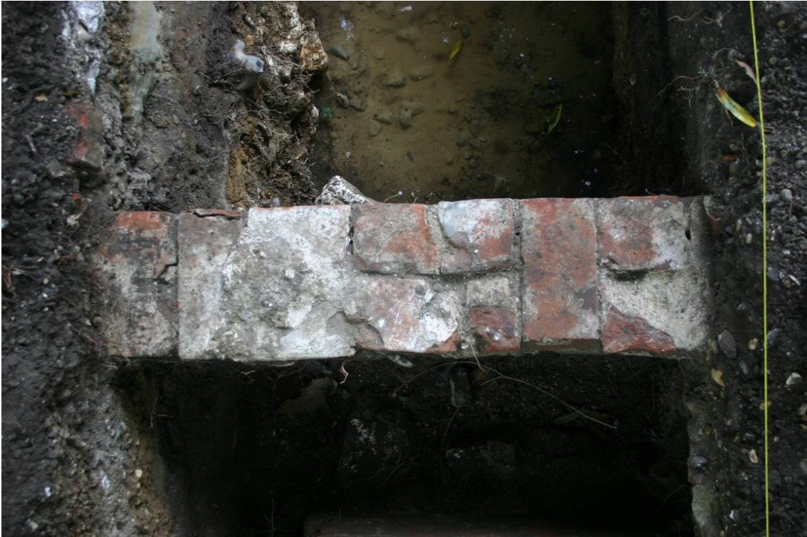
Figure 48. Foundation [B5] with east at the top of the picture.
