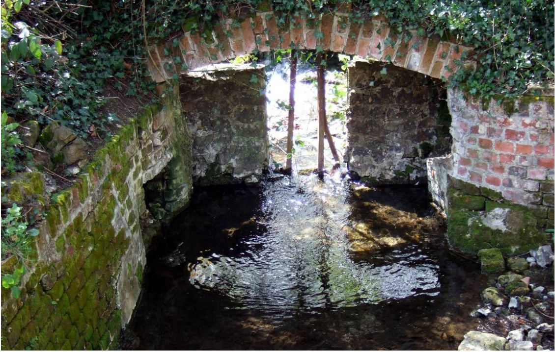
Figure 2. The downstream side of the stream entrance weir in April 2013.
