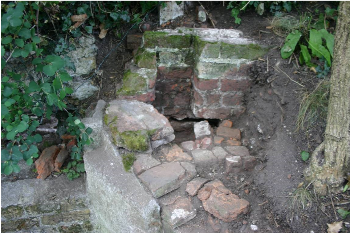
Figure 4. A brick setting for a wooden post on the garden boundary immediately south of the pond entrance weir which appears bottom left. This may once have supported a sluice gate. Looking east.
