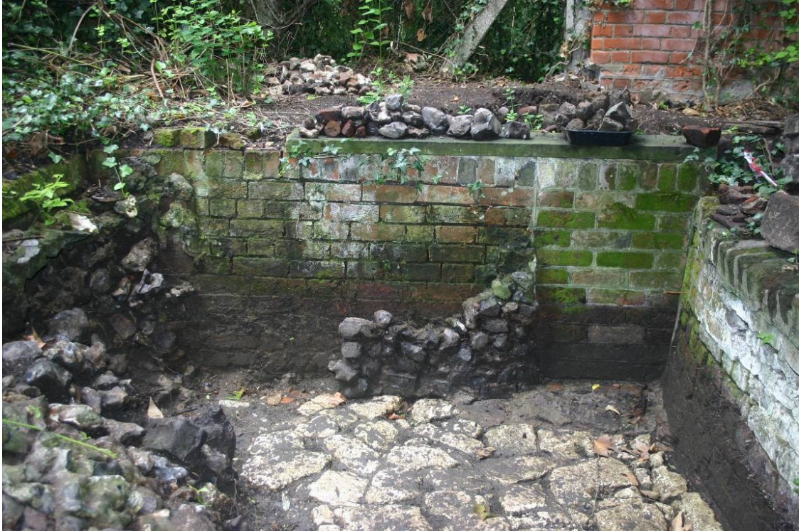
Figure 16. The north wall of the pond.
