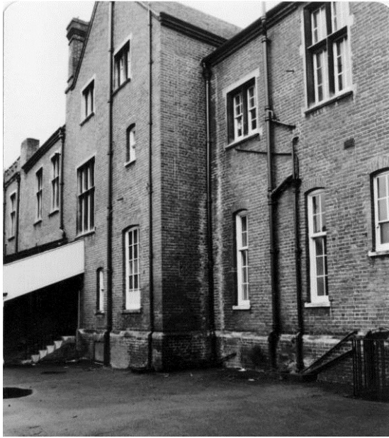
Figure 128. A bonding break on the offset of the north side of the north wing. Looking east. 10 May 1981. Note the segmental headed windows.
