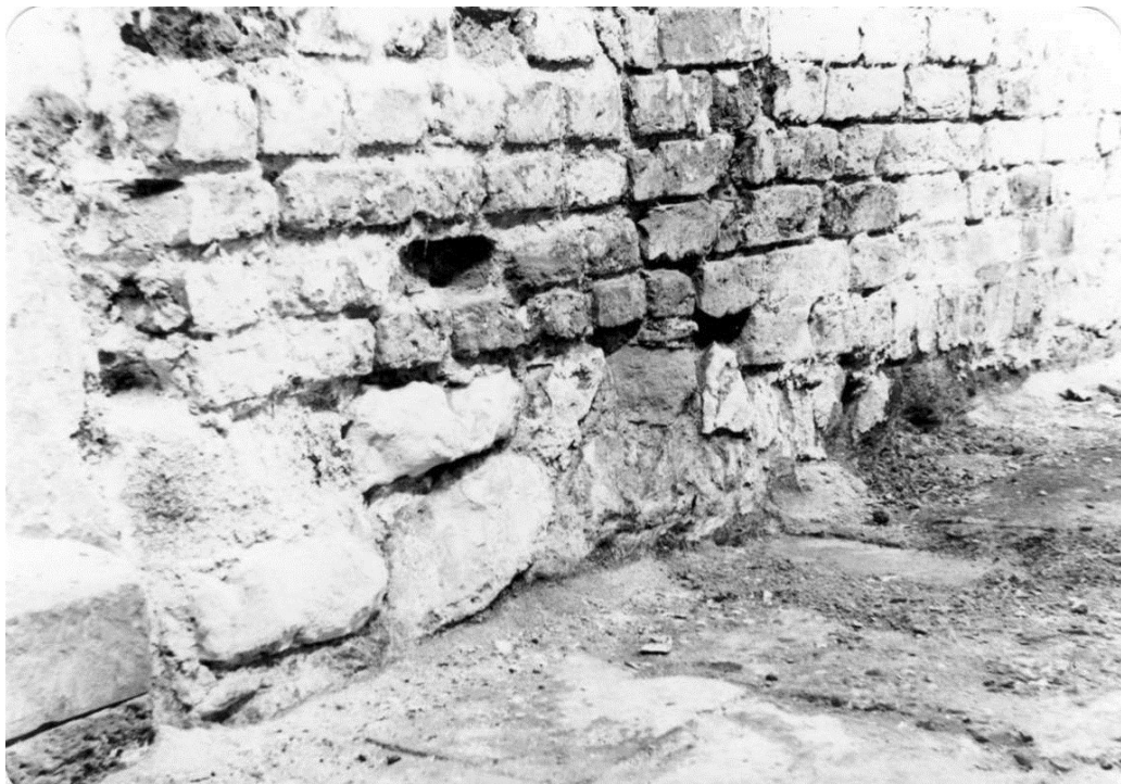
Figure 126. Stone underlying the brickwork at the bottom of the south wall of cellar 5. The door to cellar 4 is on the left.
