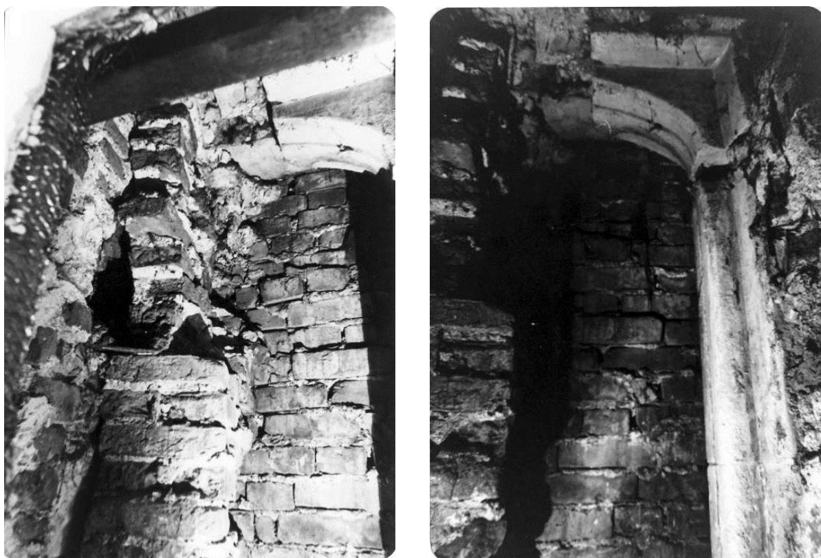
Figure 41. The Foster window showing the surviving south side and the rough brickwork installed after the north side had been removed. The windows were blocked when the house was refaced in the eighteenth century.
