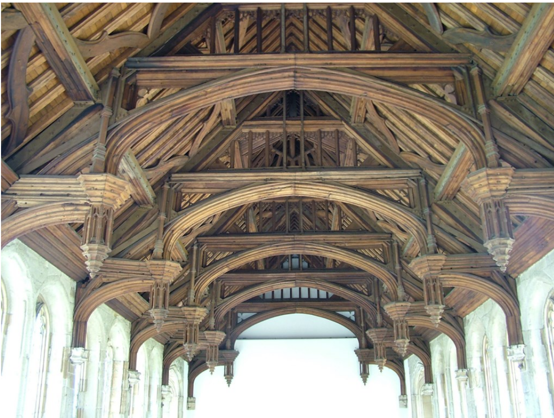
Figure 26. The Great hall roof at Eltham, Kent.
