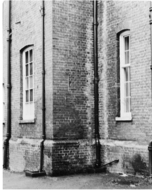
Figure 128. A bonding break on the offset of the north side of the north wing. Looking east. 10 May 1981. Note the segmental headed windows.
