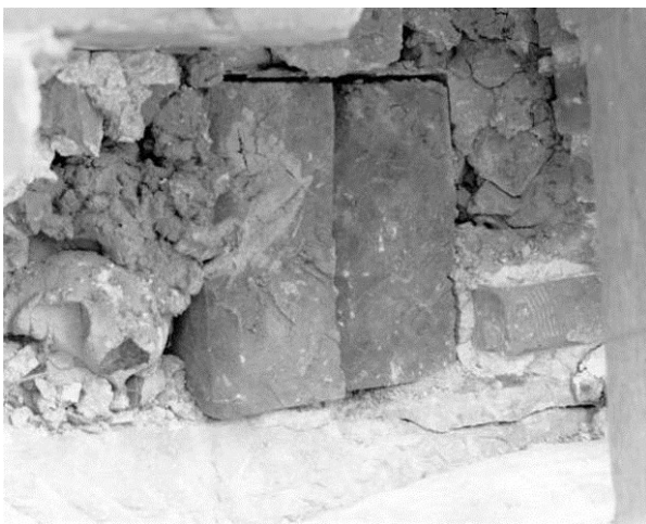
Figure 90. Cut AE – the end of two timbers resting on a stone block all embedded in the north wall of the south wing (above and below).
