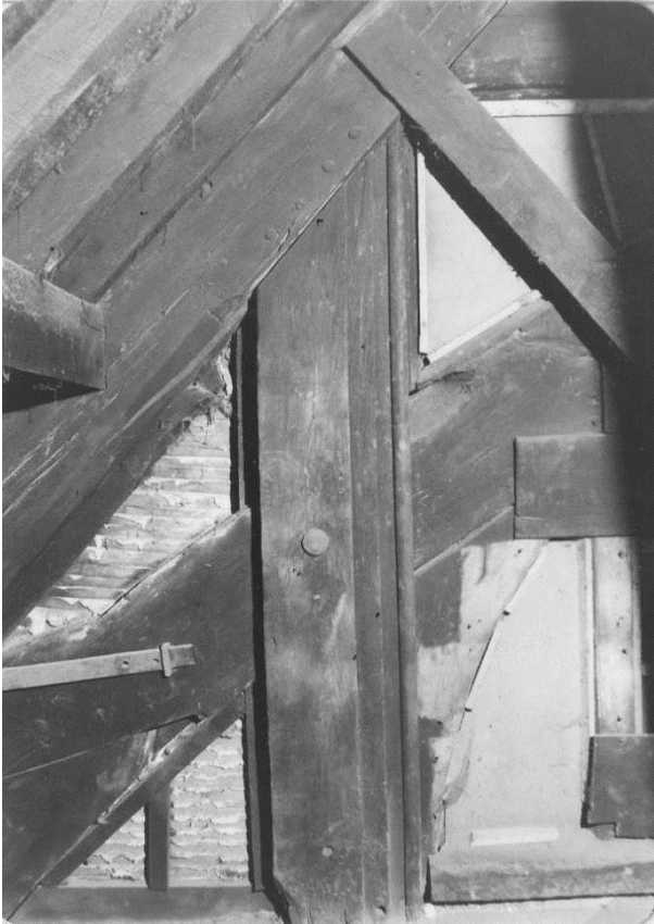
Figure 20. Truss 1, the north side of the eastern hammer-post.
