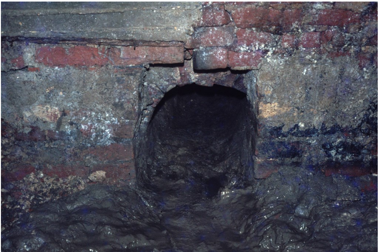
Figure 75. The main moat culvert showing entrance to side drain F1,
