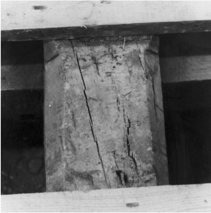
Figure 117. Upper joist 15 with lower joist 3. Looking north.
