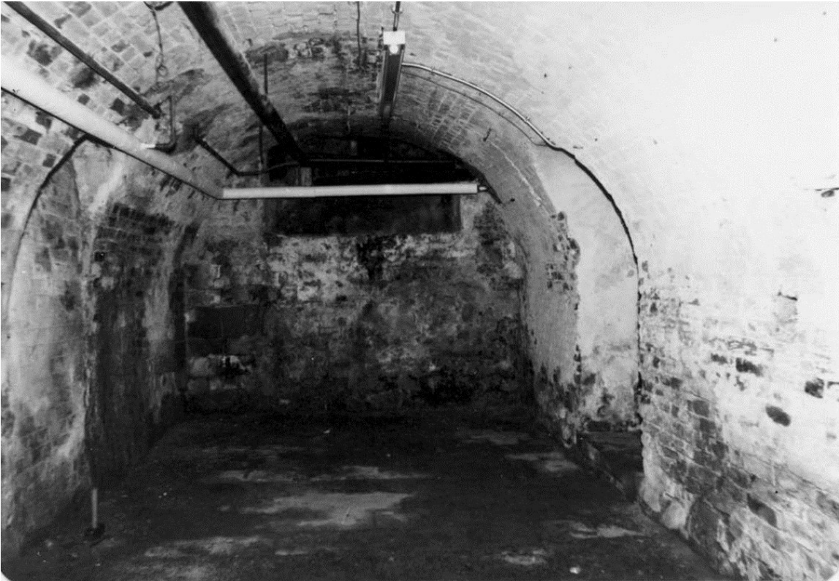
Figure 123 Cellar 5 looking east in the 1980s.
