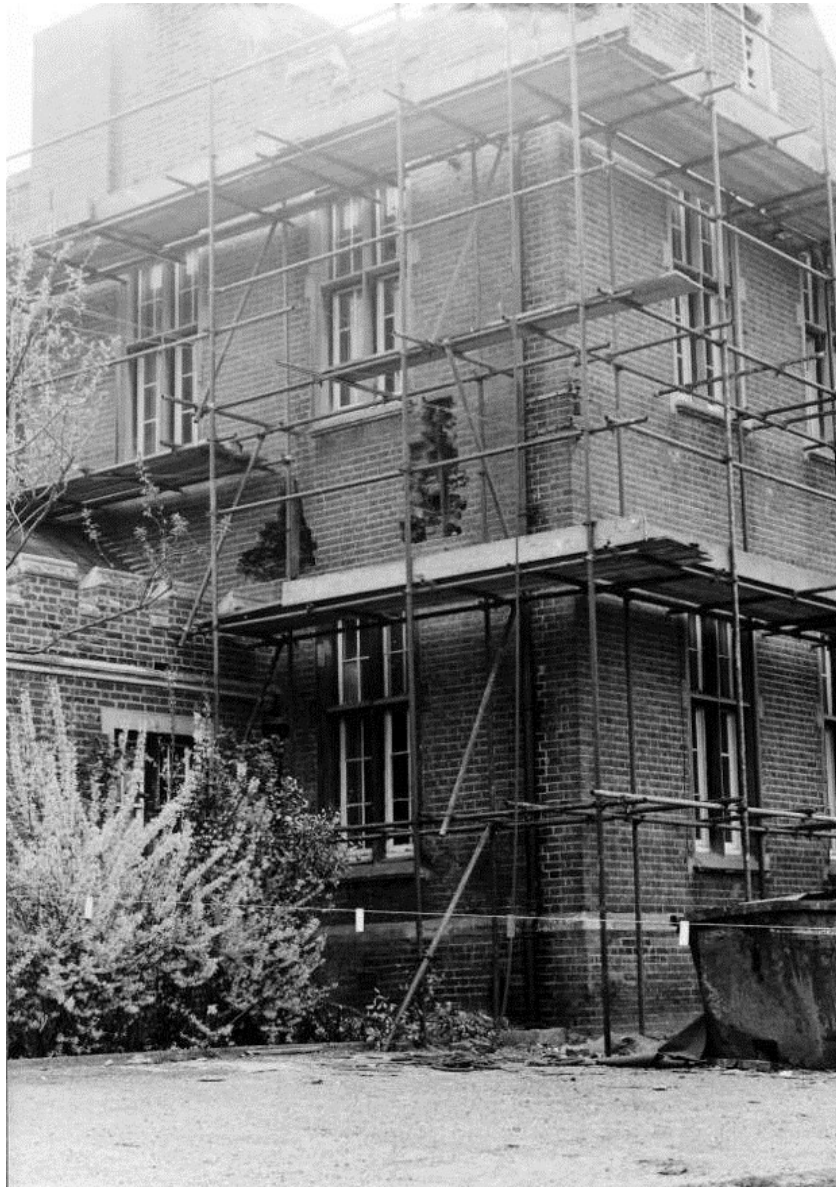
Figure 86. The two cuts AE near the northwest corner of the south wing, April 1984. The bottom of the west cut was 4.62 m above ground level.
