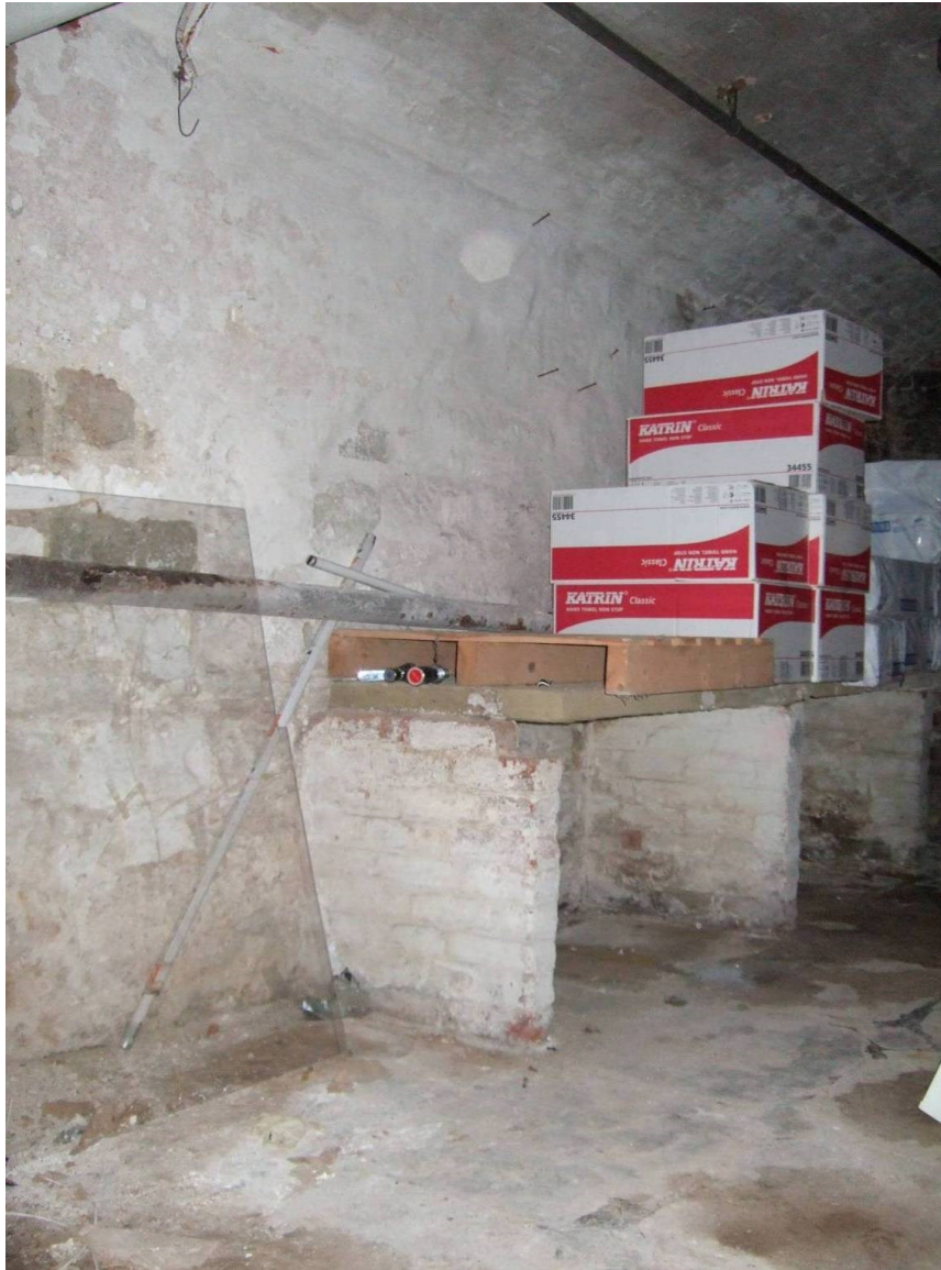
Figure 127. The western side of cellar 2 in May 2010.
