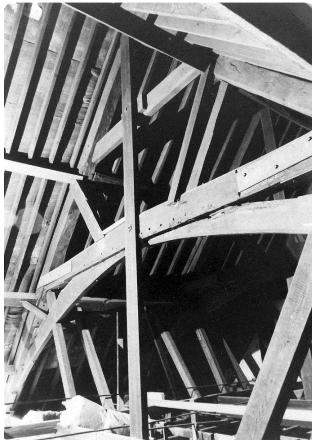
Figure 38. The service area roof showing the south side of truss 7. February 1981.
