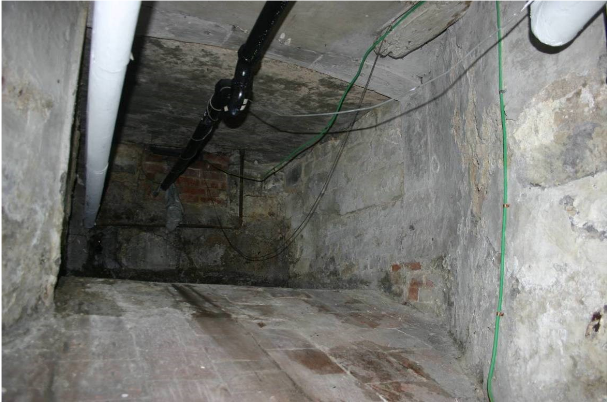
Figure 49. The barrel chute on the west side of cellar 6 in August 2007.
