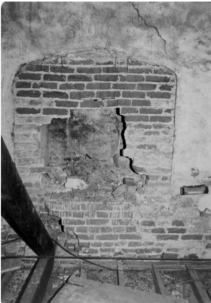
Figure 132. The fireplace in the chimney stack on the north wall of the hall in 1981 after the brick blocking had partially collapsed. Note the U-shaped ledge at the back of the fireplace.
