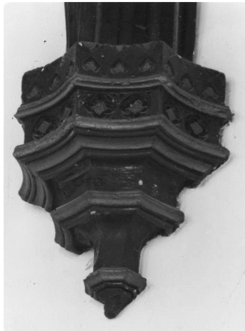
Figure 22. The corbel on the east side of truss 2.
