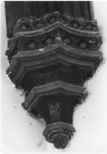
Figure 21. The corbel on the east side of truss 1.
