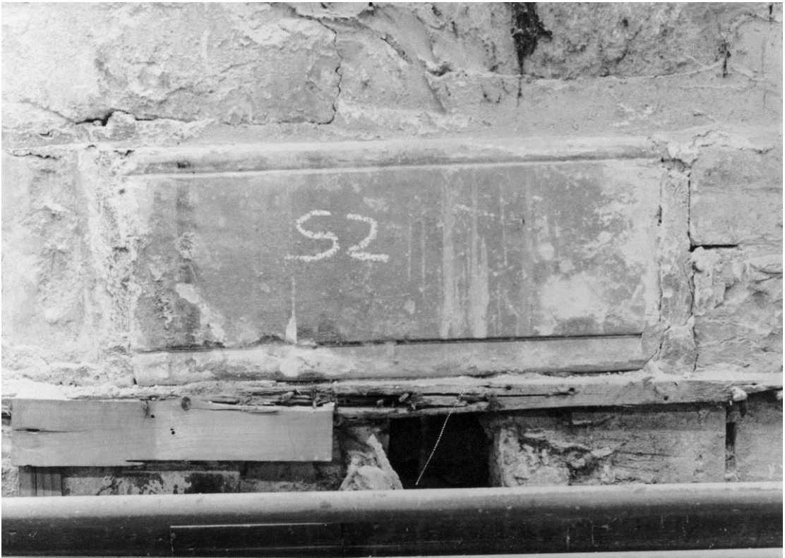
SB 102 in situ in the gymnasium wall.
