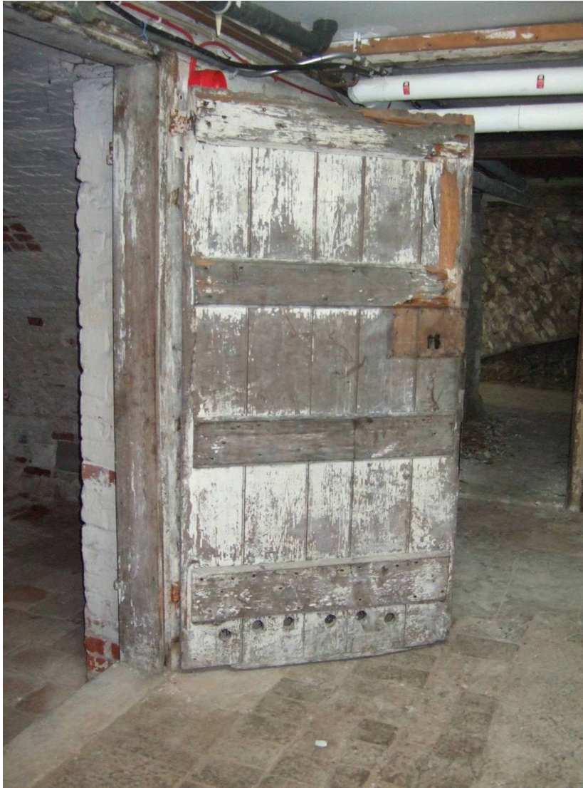
Figure 51. The door between cellar 6 (right) and cellar 7 (left) in May 2010.
