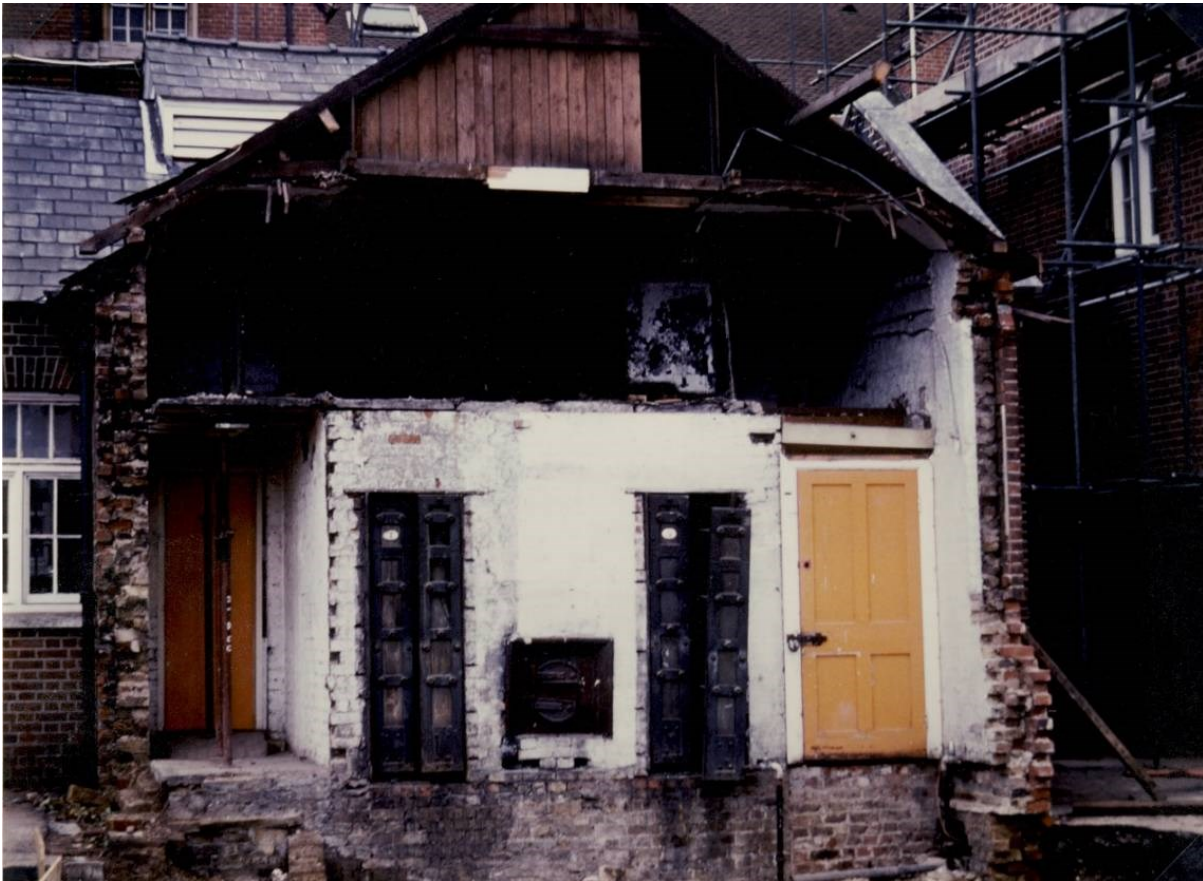
Figure 8. The former laundry in 1983. The north end of the building has been demolished. Note the ends of the drying racks with the massive cast iron fore grate between them. The wood at the top of roof enclosed a water tank.
