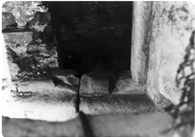
Figure 43. The bottom of the window.
