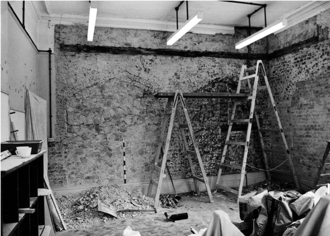
Figure 99. Blocked arches exposed in the east wall of room 134 on 1 September 1986.
