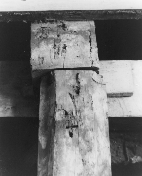
Figure 111. Upper floor joist 5 with lower floor joist 3 looking south.
