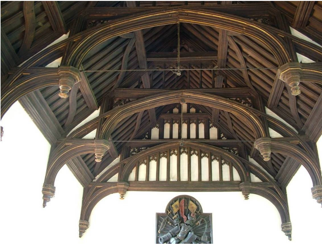
Figure 25. The hall roof at Beddington looking north
