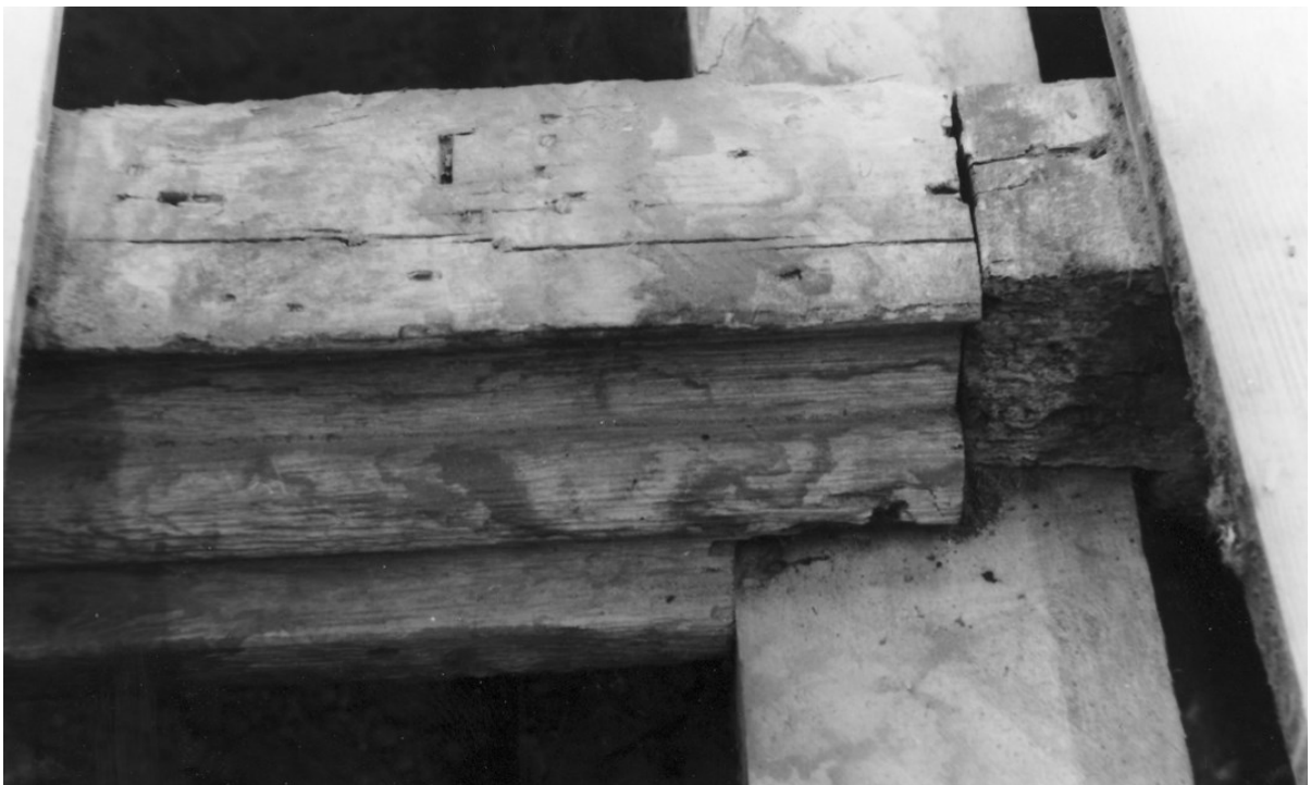
Figure 114. Upper joist 9 with lower joist 2 on the right. Looking east.
