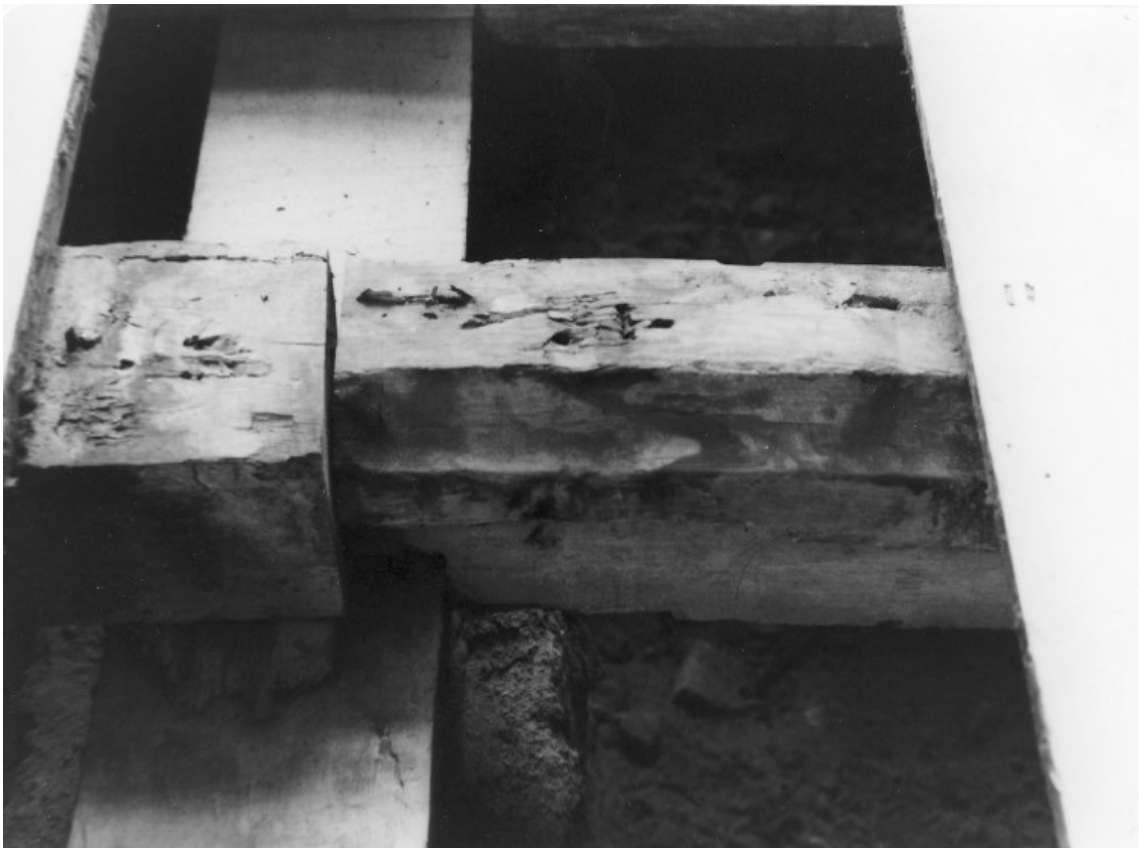
Figure 110. Upper floor joist 5 with lower joist 3. Looking west.
