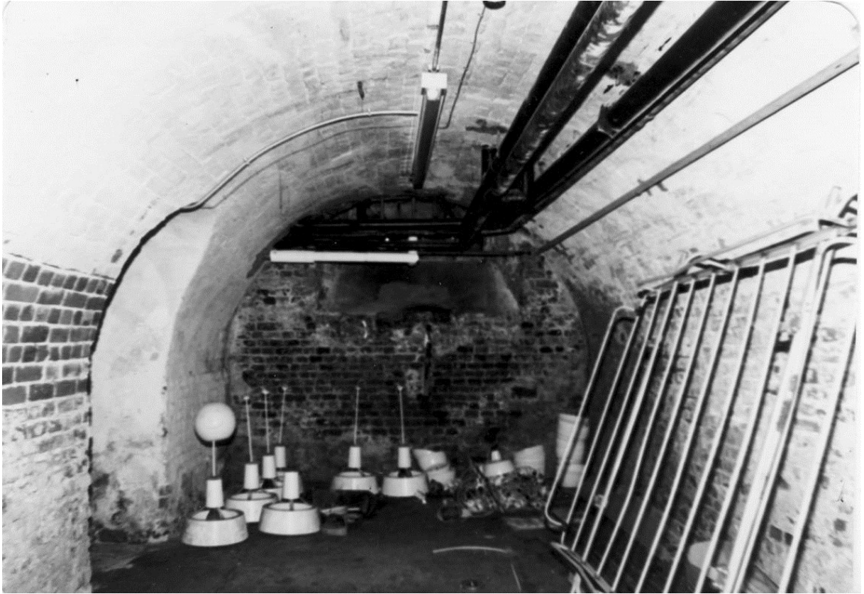
Figure 121. Cellar 4 looking east in the 1980s. Note the contrast between the eighteenth century bricks in the vault and the Tudor ones in the end wall which is the eastern outer wall of the north wing. The door to cellar 5 is on the left.
