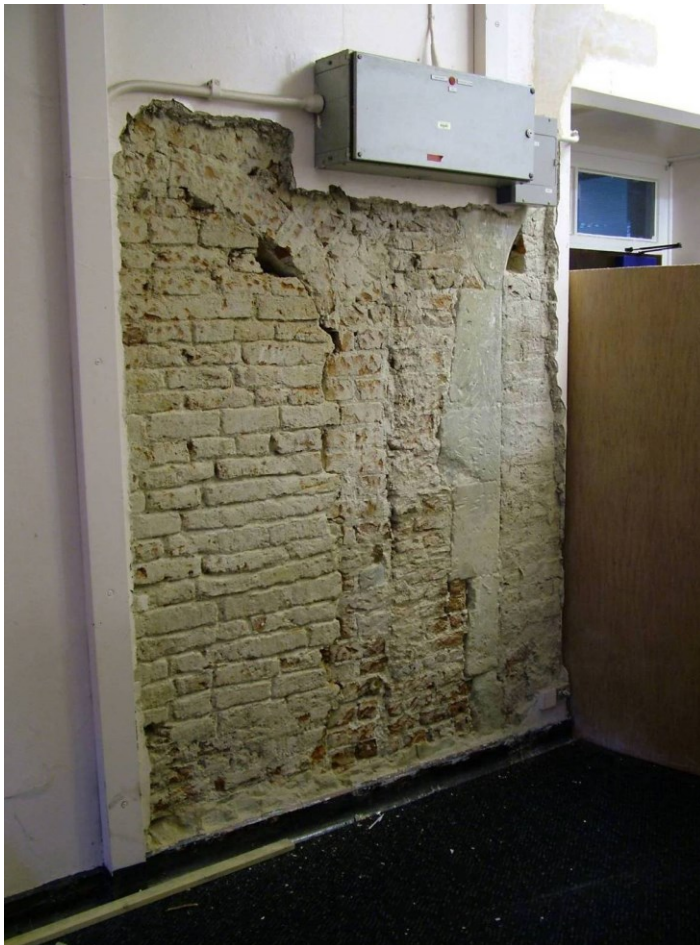
Figure 47. Exposed brickwork in the hall corridor [DH].
