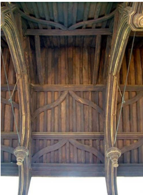
Figure 16. The east side of bay 2.
