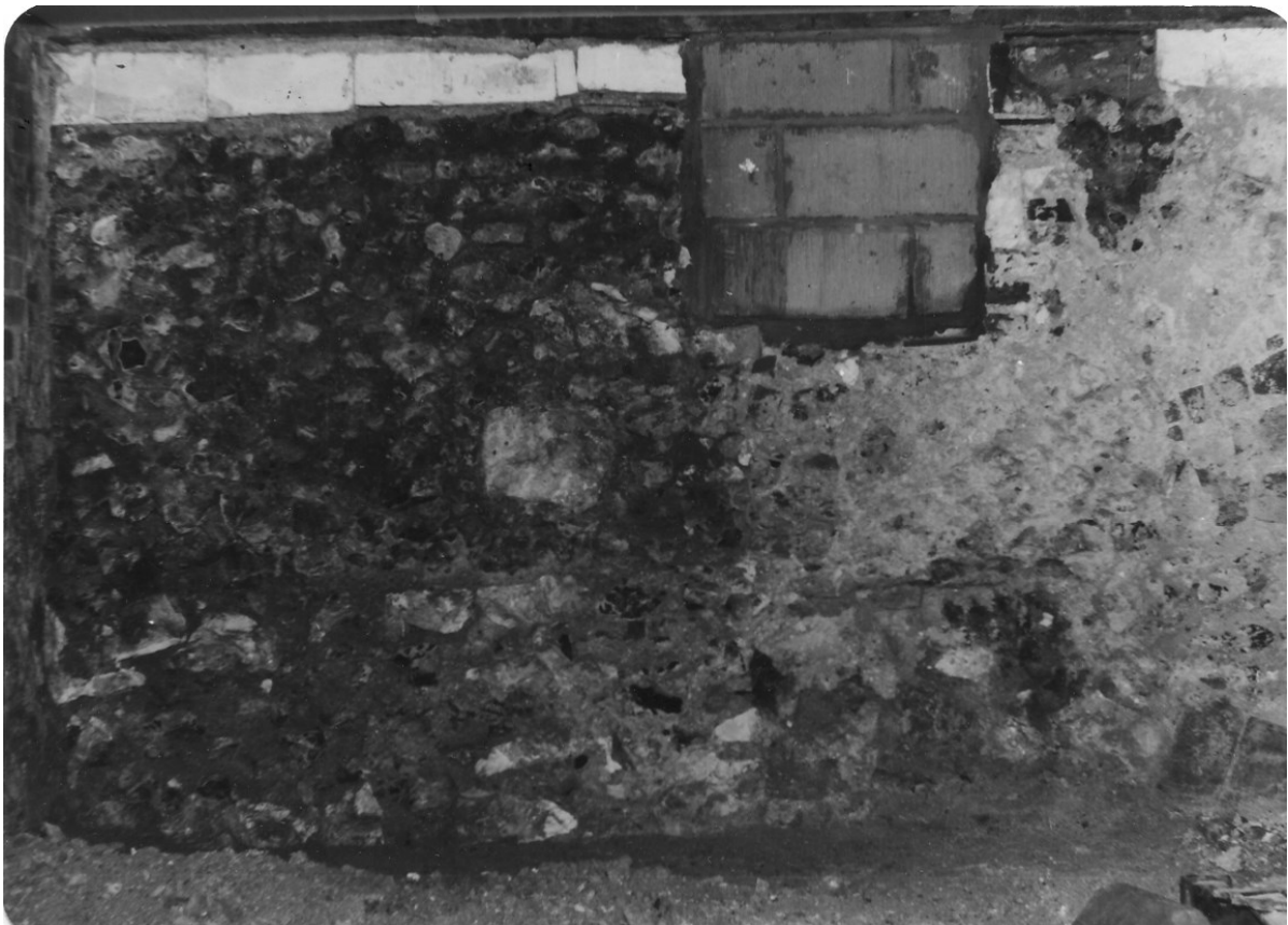
Figure 62. The south wall of cellar 8.
