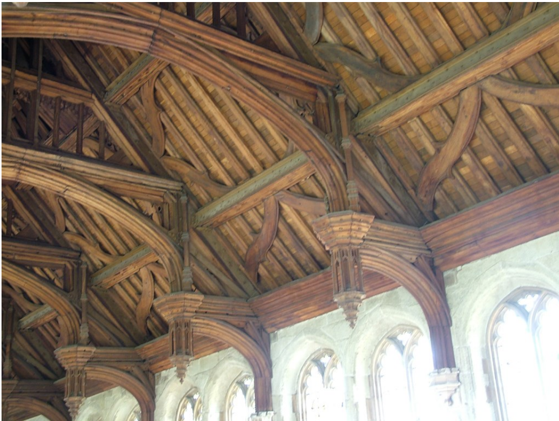
Figure 28. The Great hall roof at Eltham, Kent.
