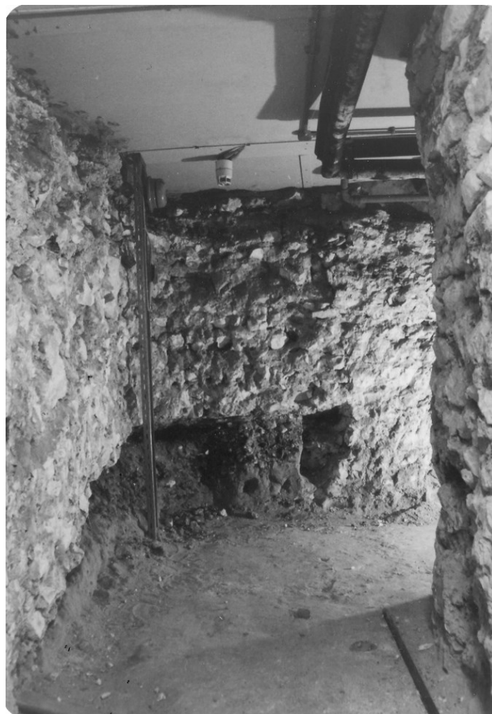
Figure 68. Passage 2 looking west showing the chalk rubble kitchen foundations, the vault and its earth fill.
