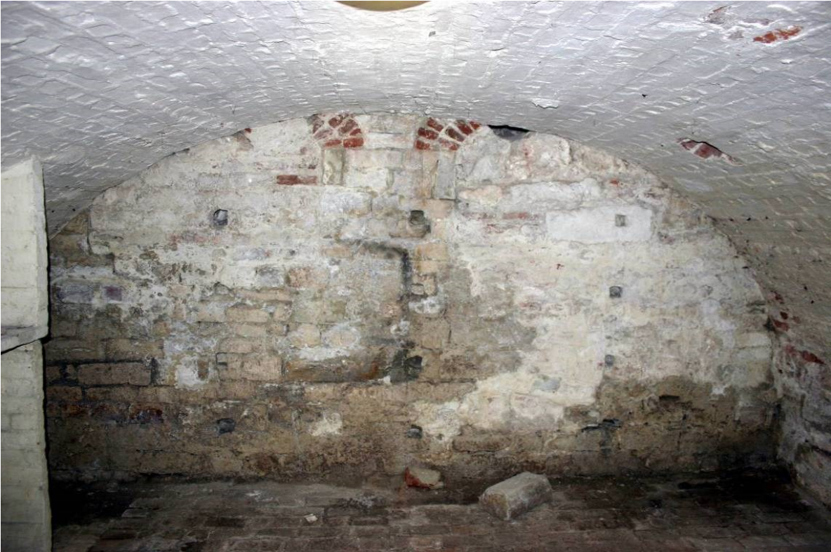
Figure 53. The east wall of cellar 7 in August 2007.
