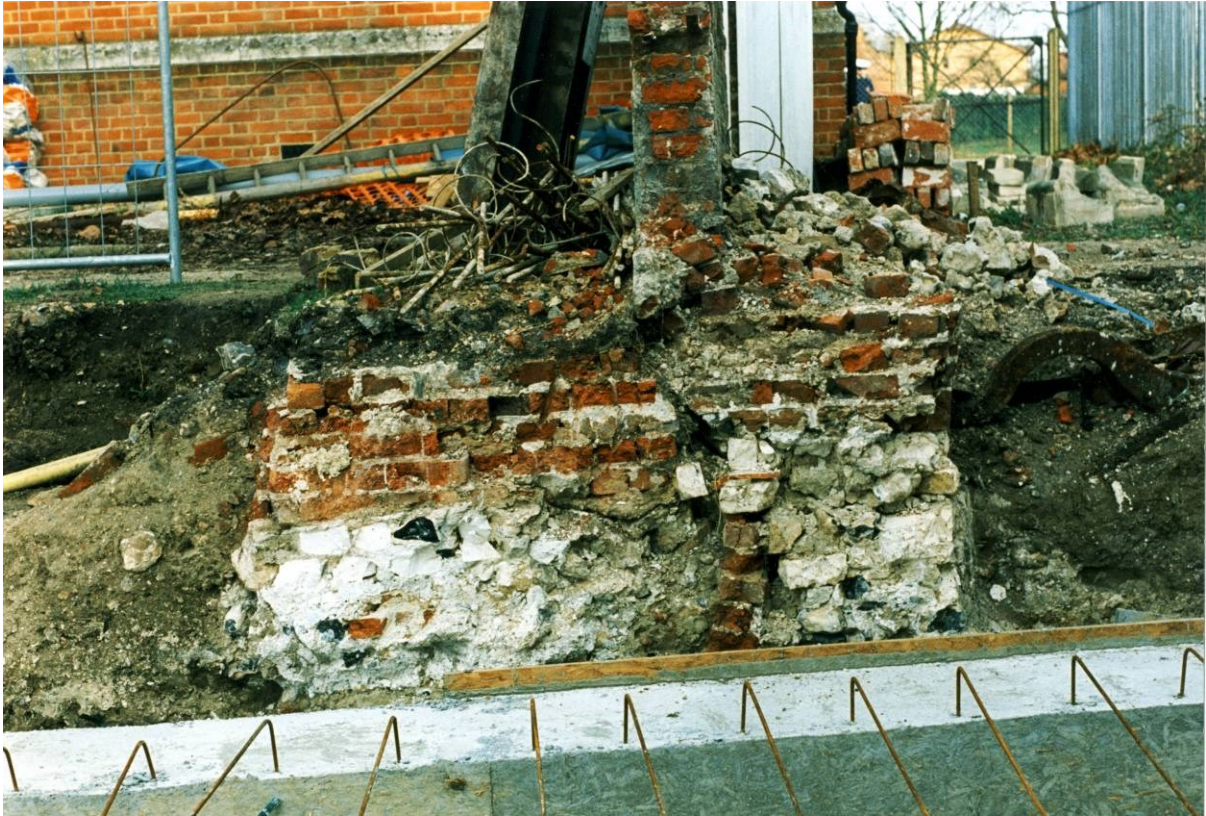
Figure 56. Section of the moat wall exposed in the foundation trench for the church extension. Looking east with the school gymnasium in the background. (For interpretation see figure 57).
