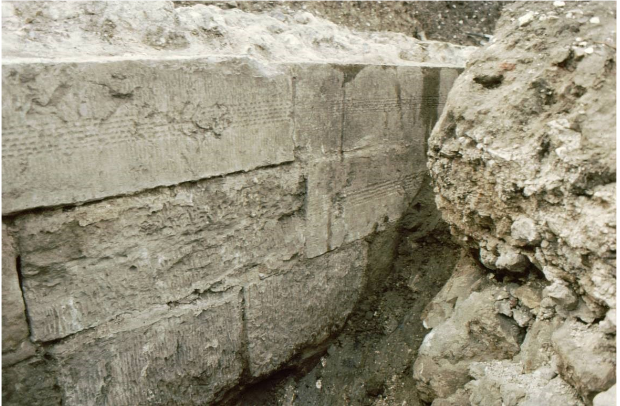
Figure 35. The outer face of the moat wall in trench CA.
