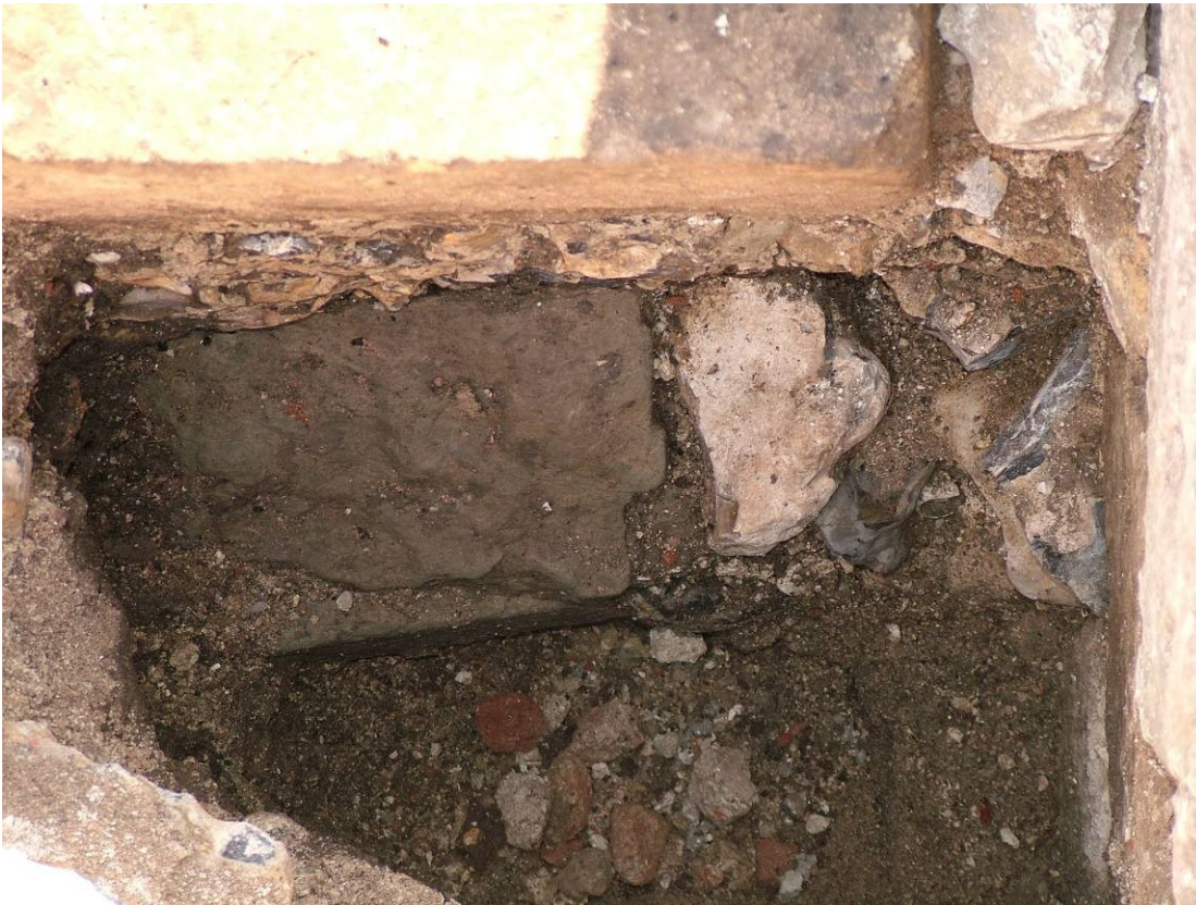
Figure 102. Looking down on the offset on the south side of the moat wall [CEZ24]. The abutment [CEZ23] on the right.
