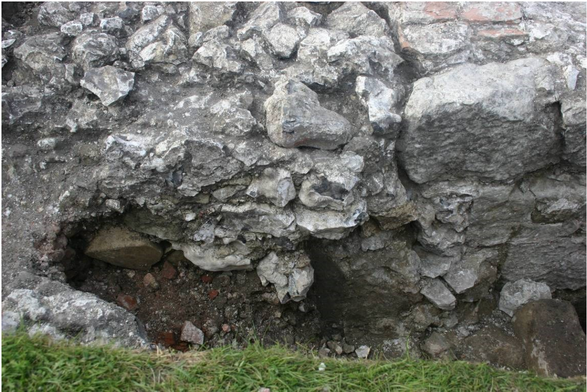
Figure 96. The wall [CEZ33] with [CEZ23] the right and the top of the southward running wall [CEZ24] just visible bottom right.
