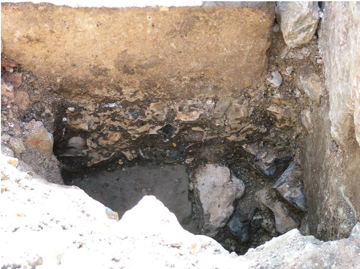
Figure 101. The south side of the moat wall [CEZ24] showing the flint bonded into the abutment wall [CEZ23].
