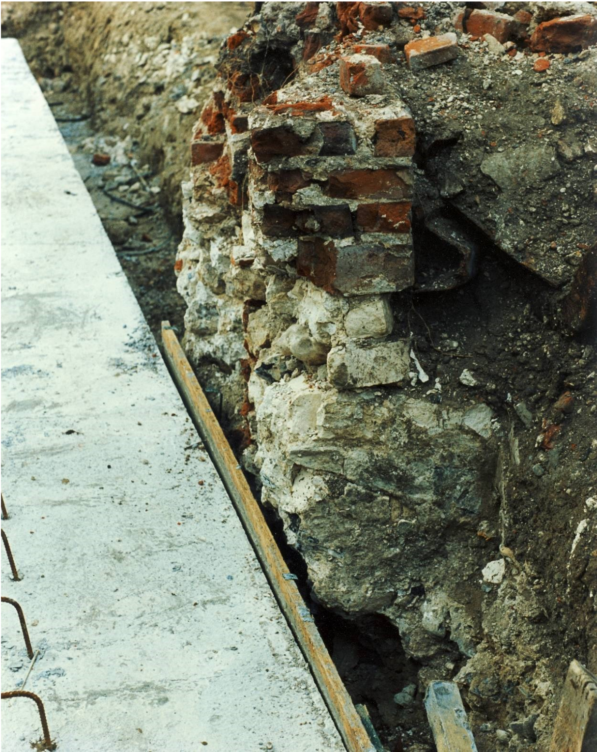
Figure 58. The stone and mortar foundation of the churchyard (moat) wall below the brick foundation of the wall connecting the churchyard to the south wing. Looking north.
