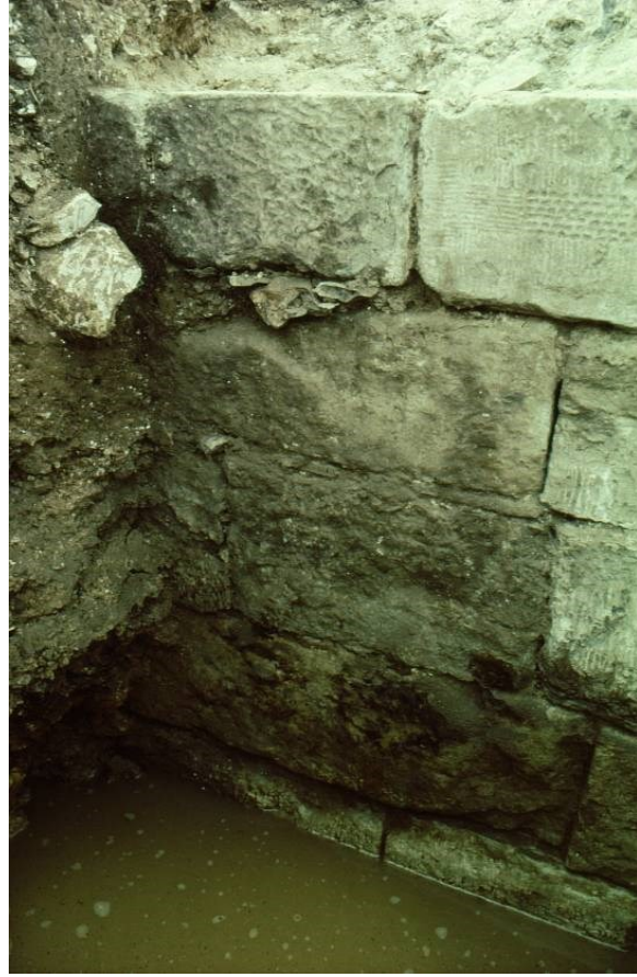
Figure 33. The moat wall in CA, looking southwest.
