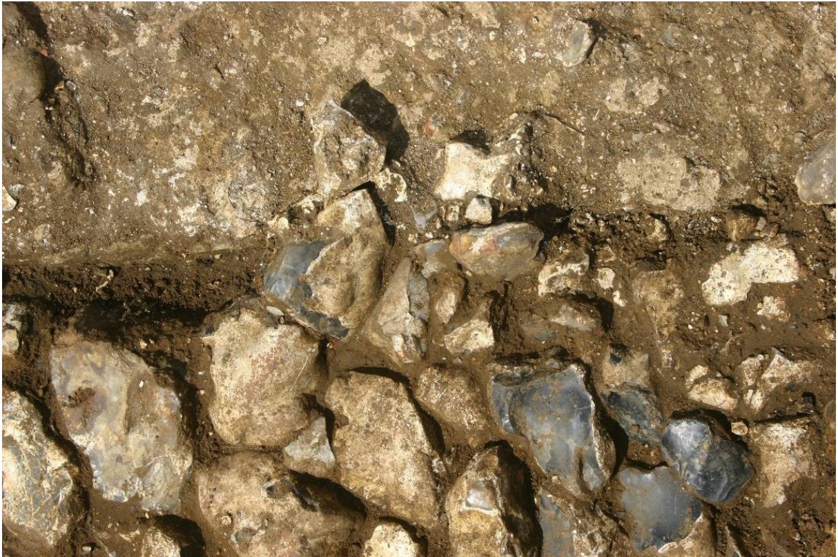
Figure 90. The cobbled surface [CEZ18] lapping over the eastern edge of the abutment.
