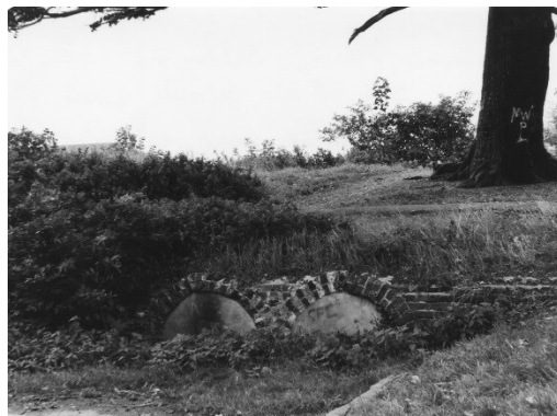
Figure 18. The cascade culverts in 1987.
