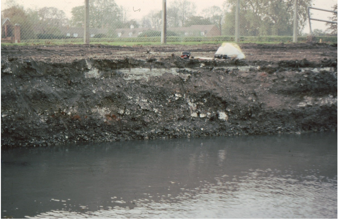
Figure 31. Section FE on the west side of the realigned channel next to the former swimming pool.
