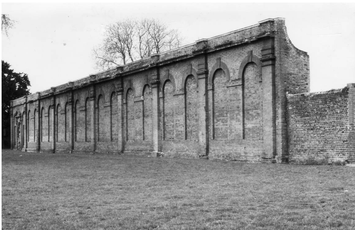
Figure 12. The north side of the Orangery wall from the west end.
