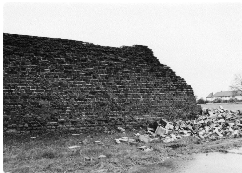
Figure 8. The remains of the wall between the north gate and river on 3 May 1981. Note the bond break adjacent to the gate pier.
