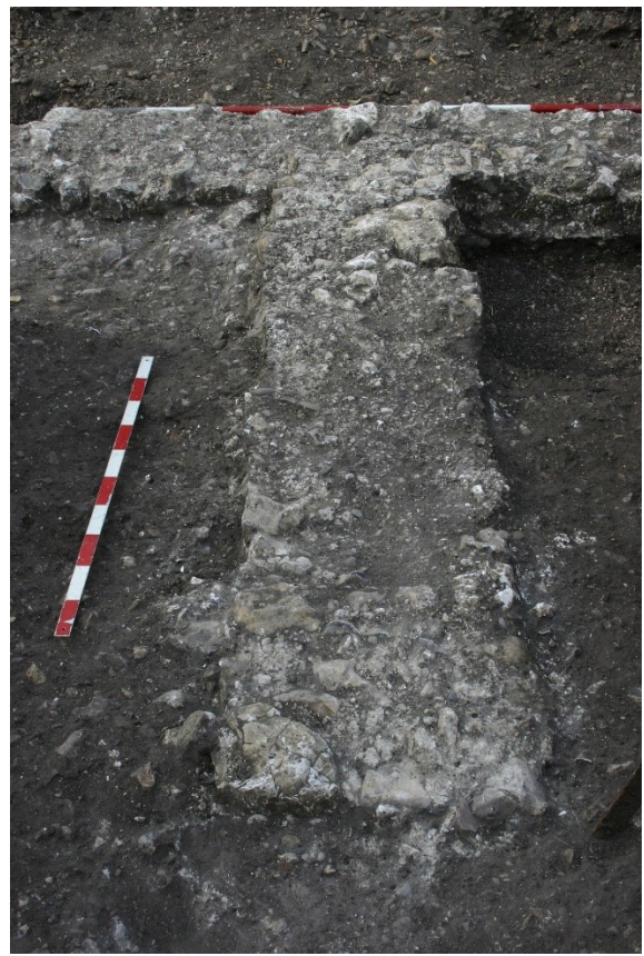
Figure 18. Trench A: foundation [5] and projection P4 looking north.
