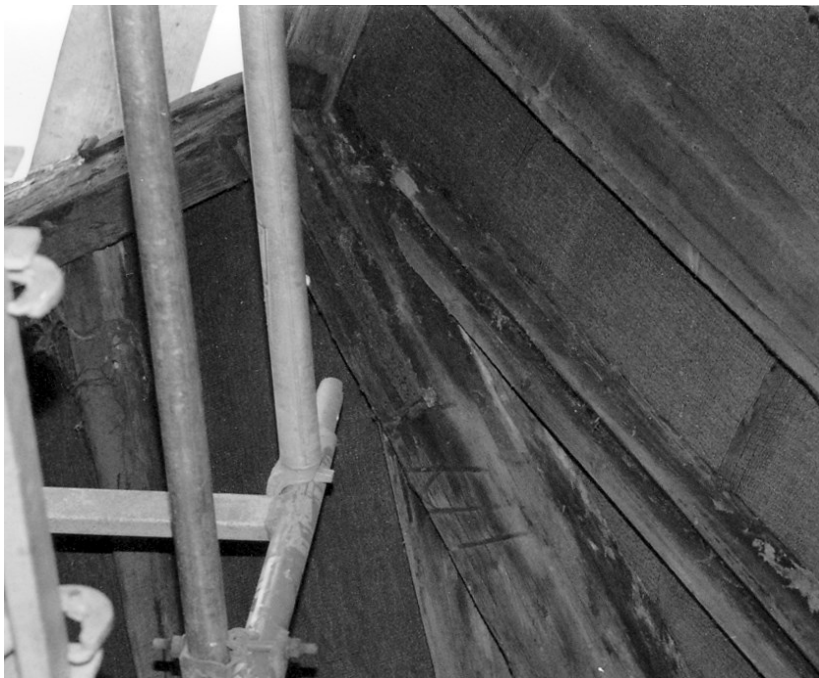
Figure 35. The carpenter's mark on the top of principal rafter 1.
