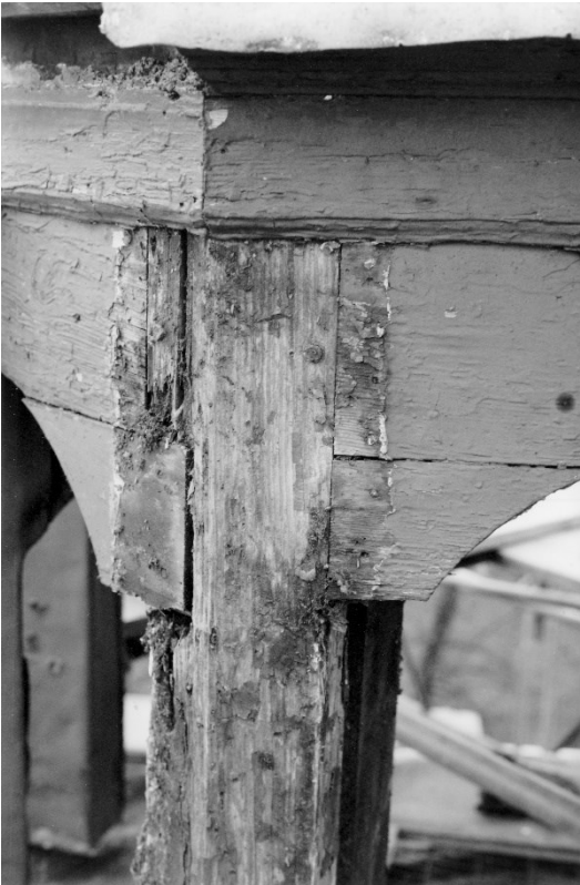
Figures 7 (left) and 8 (right). The top of the turret showing the junction between the columns and the boards forming the arch. Note the use of nails.
