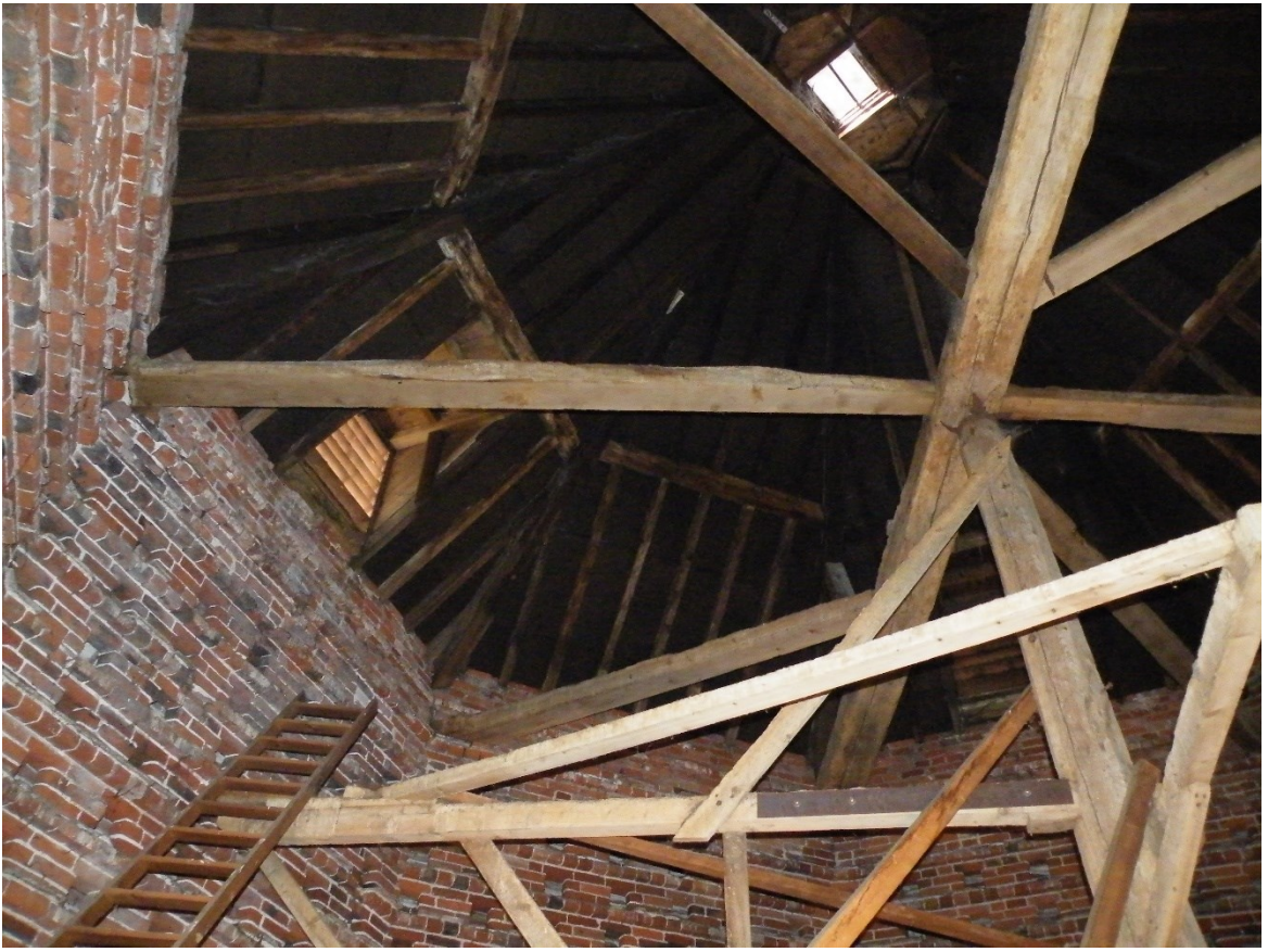
Figure 17. The south side of the roof looking west.
