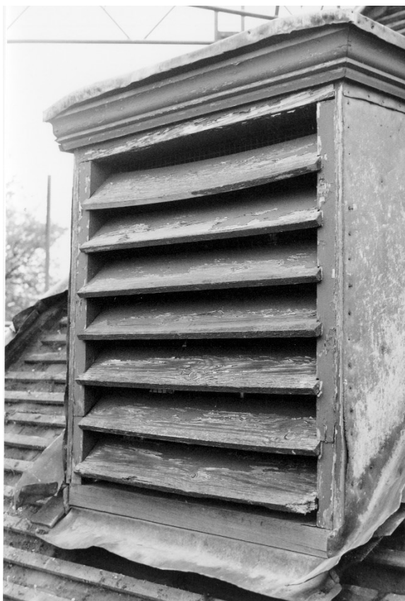
Figure 25. The front of the southeast ventilator.
