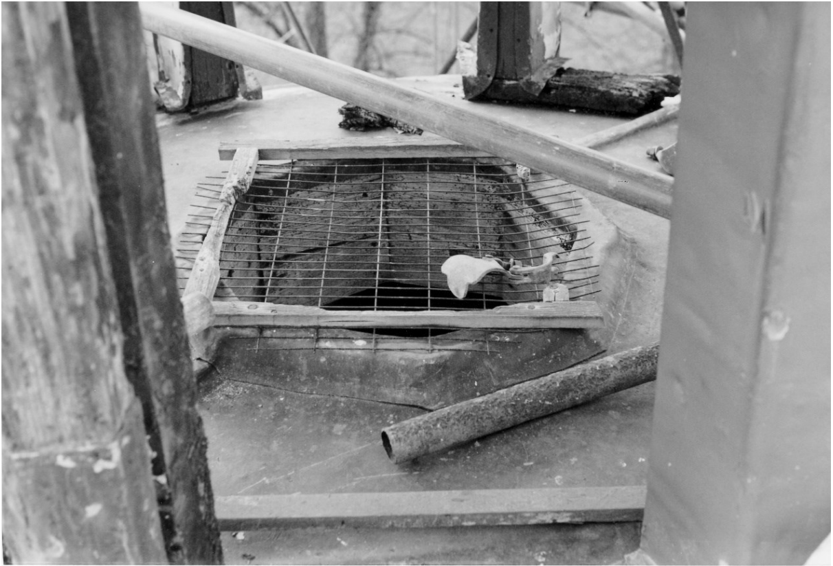
Figure 13. The floor of the turret showing the wired-off entrance where the birds came in and out
