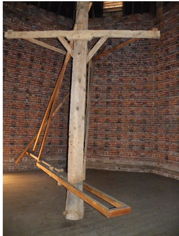
Figure 46. The bridging beam with the base of the potence and the top of the central post.
