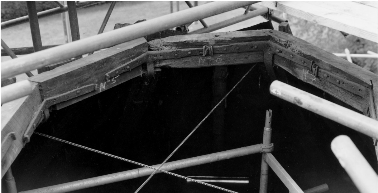
Figure 22. The ring beam showing the mixture of old and new timbers.
