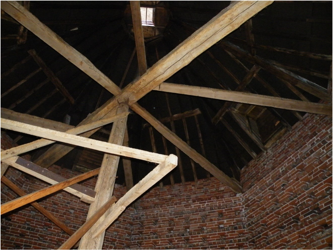
Figure 18. The north side of the roof looking northwest.
