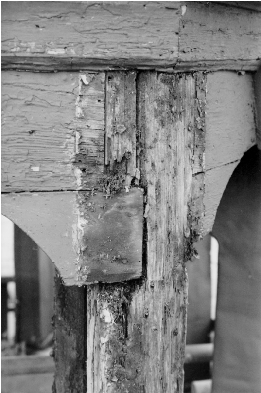
Figures 7 (left) and 8 (right). The top of the turret showing the junction between the columns and the boards forming the arch. Note the use of nails.
