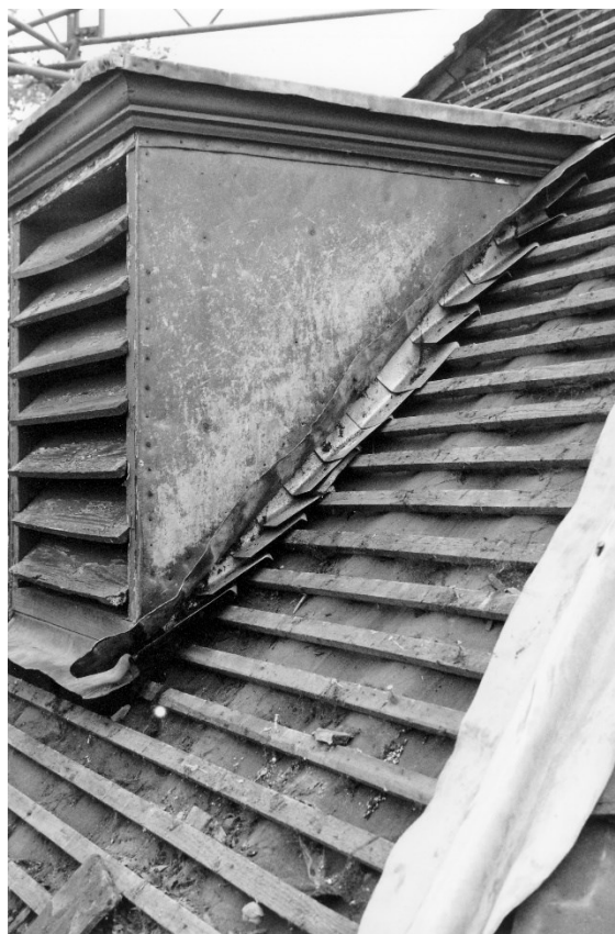
Figure 26. The north side of the southeast ventilator.
