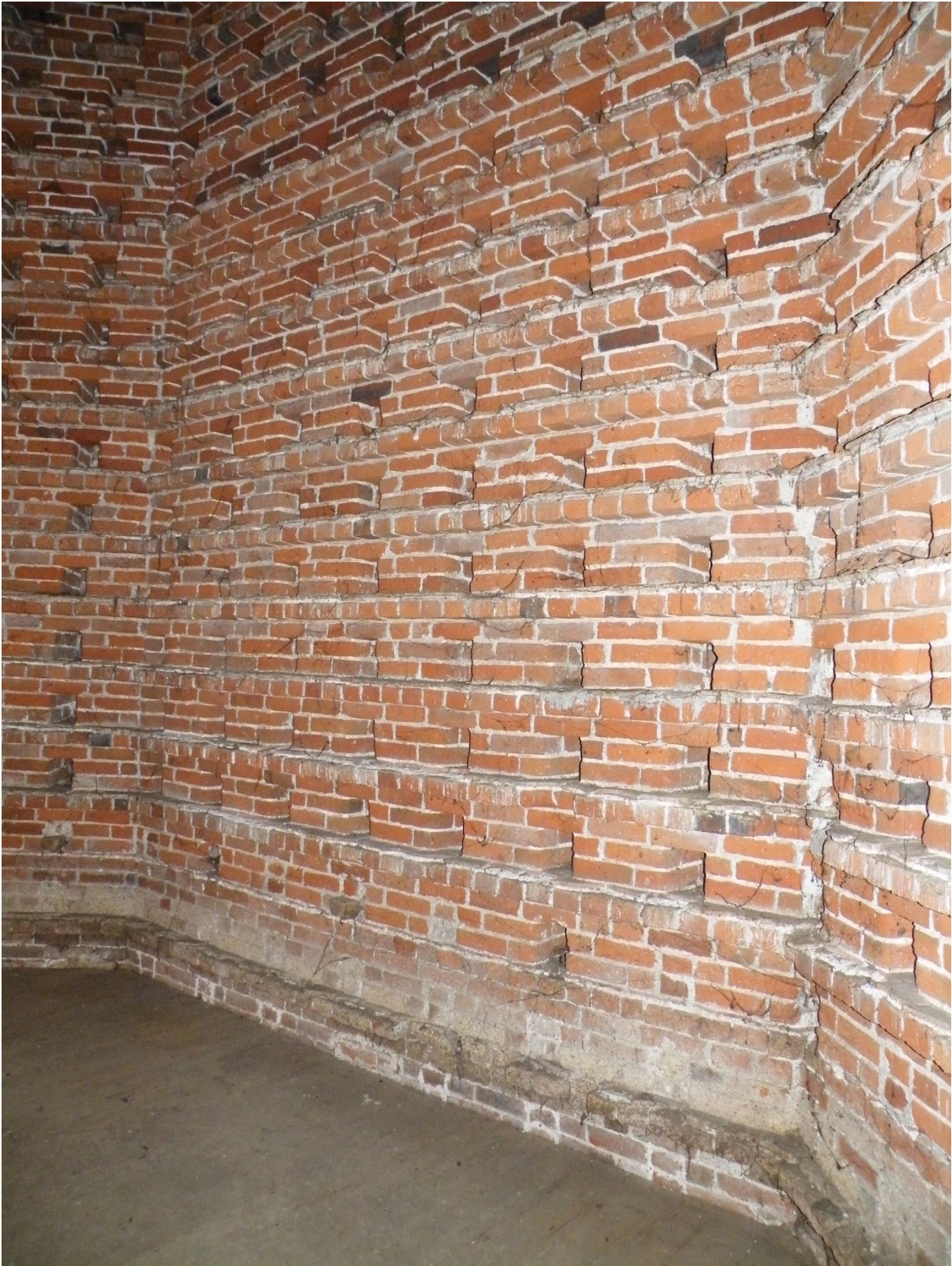
Figure 38. The nesting boxes inside the dovecote.
