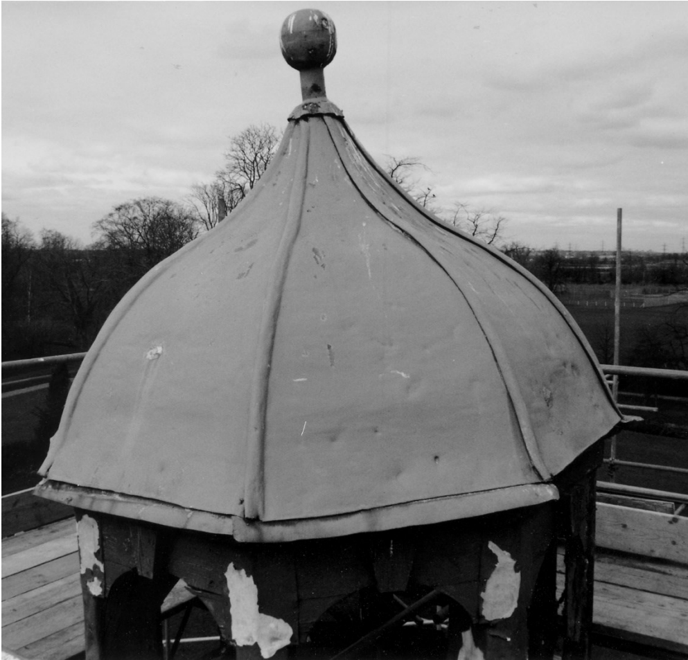
Figure 2. The roof of the turret looking northwest.
