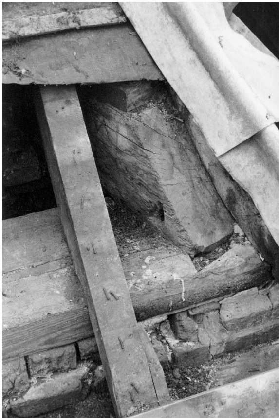
Figure 30. The north side of corner 6.
