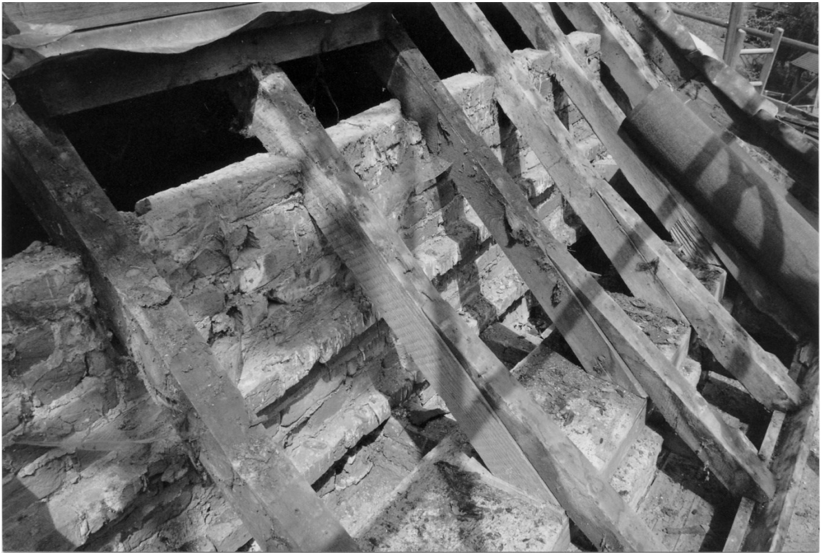
Figure 43. The back of the front wall of the nesting boxes.
