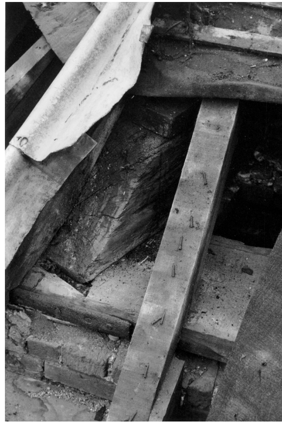
Figure 31. The south side of corner 6.
