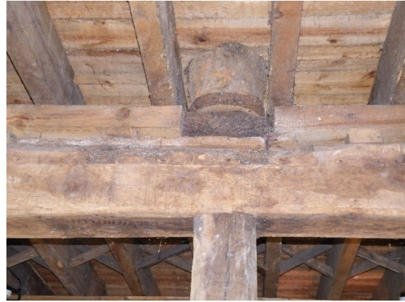
Figure 46. The bridging beam with the base of the potence and the top of the central post.
