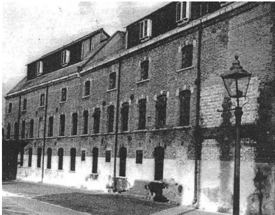
Drying lofts with later clerestory. (BP photo archive – M Ball).
