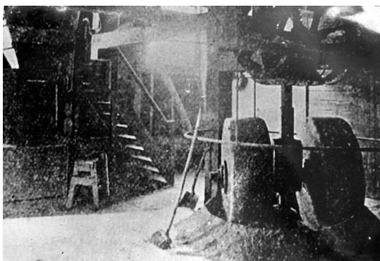
Edge runner mill for coarse grinding. (SLSC.)
