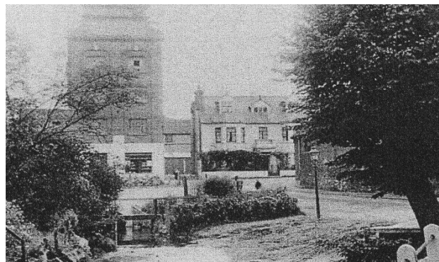
Wandle Flour Mills and Mill House,
