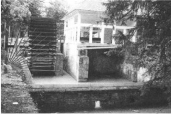
Upper Mill was rebuilt as an electricity generator. 2004 view. Photo by D E Bradford.
