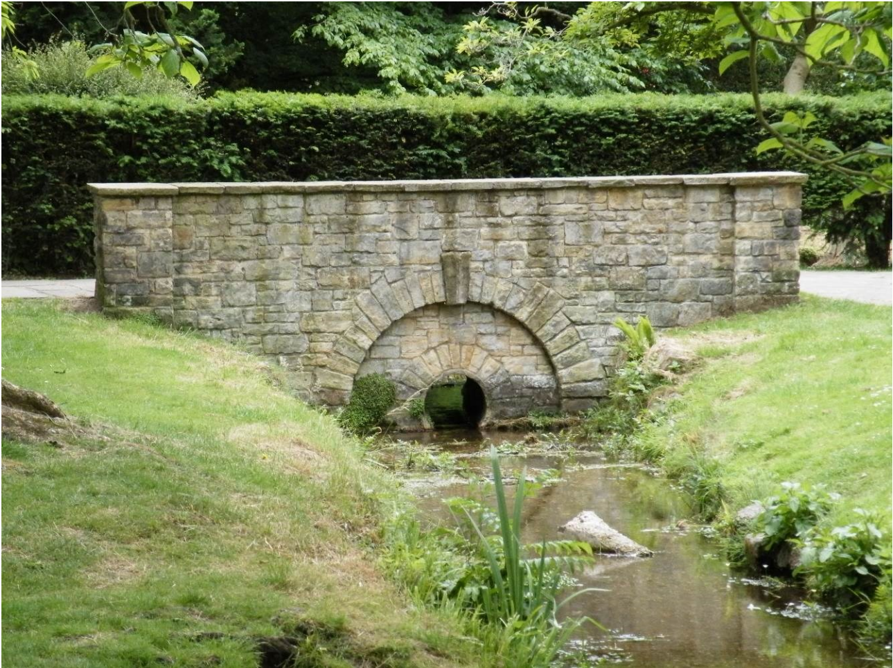
Figure 116. The upstream side of bridge F looking south in 2013.
