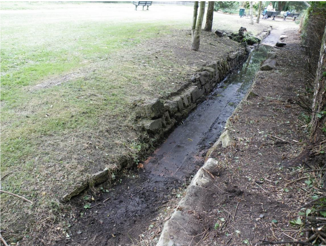
Figure 120. The remains of the fernery looking west in 2015.
