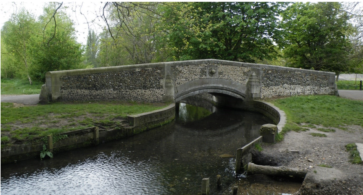
Figure 29. The upstream side of the flint bridge in 2019.
