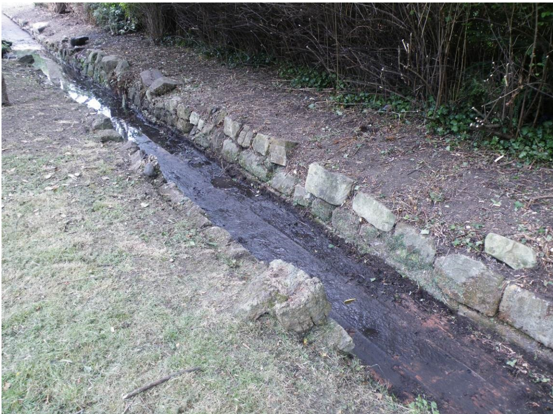
Figure 122. The rock work along the north side in 2015.
