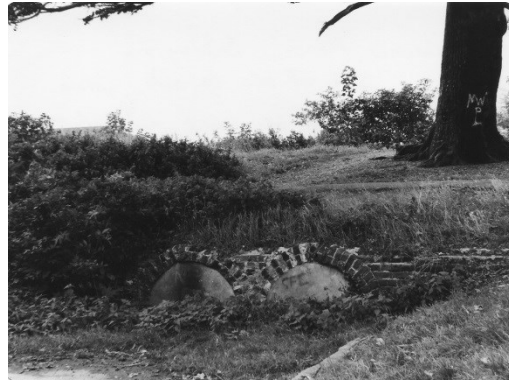
Figure 75. The cascade culverts in 1987.
