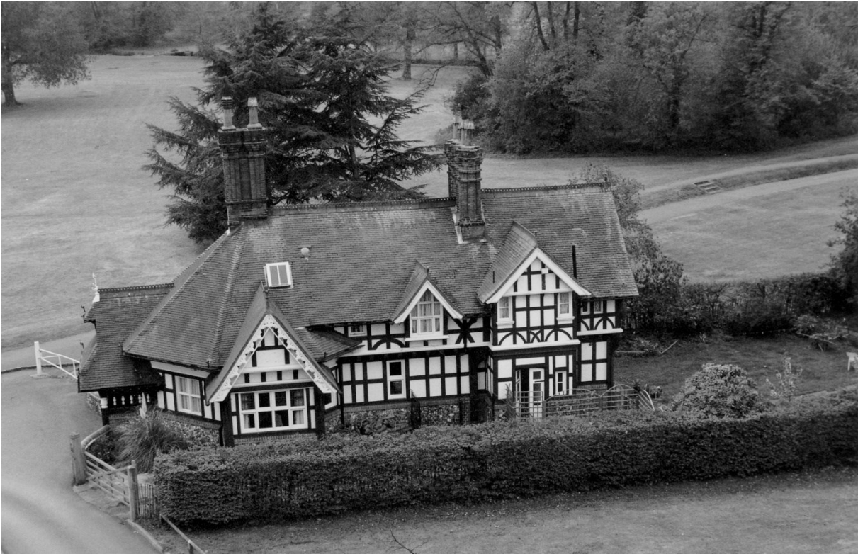
Figure 38. East Lodge photographed from the scaffolding used to repair the dovecote in 1987.
