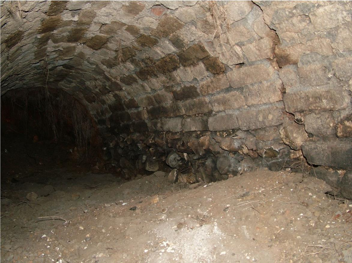
Figure 212. The south side of the culvert in 2004 with the crack at the end of section 3.
