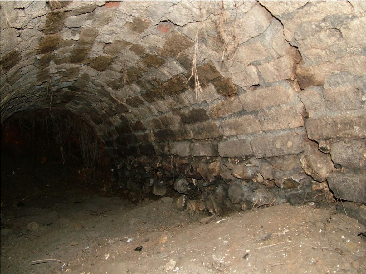
Figure 215. The south side of culvert section 4 in 2004 with the crack in section 3 on the right.
