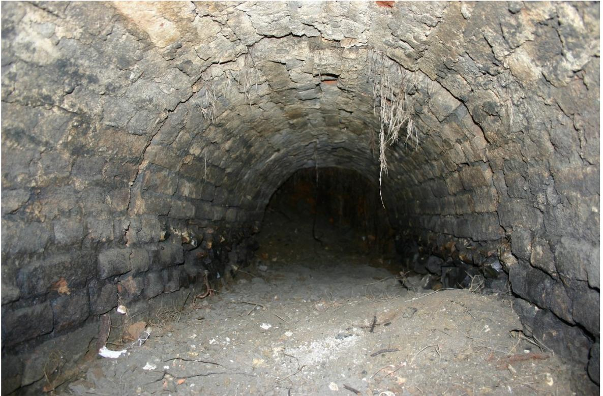
Figure 210. Looking from culvert section 3 into culvert section 4 in 2004, showing the crack in the roof.
