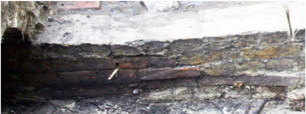
Figure 206. Detail showing the hack mark on one of the red bricks in the older lower part of the north wall of culvert section 2.
