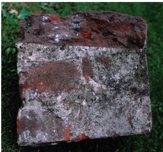
Figure 226. Brick clump <129> from [CW3/5]. Note the wedge shaped mortar to start the turn of an arch.
