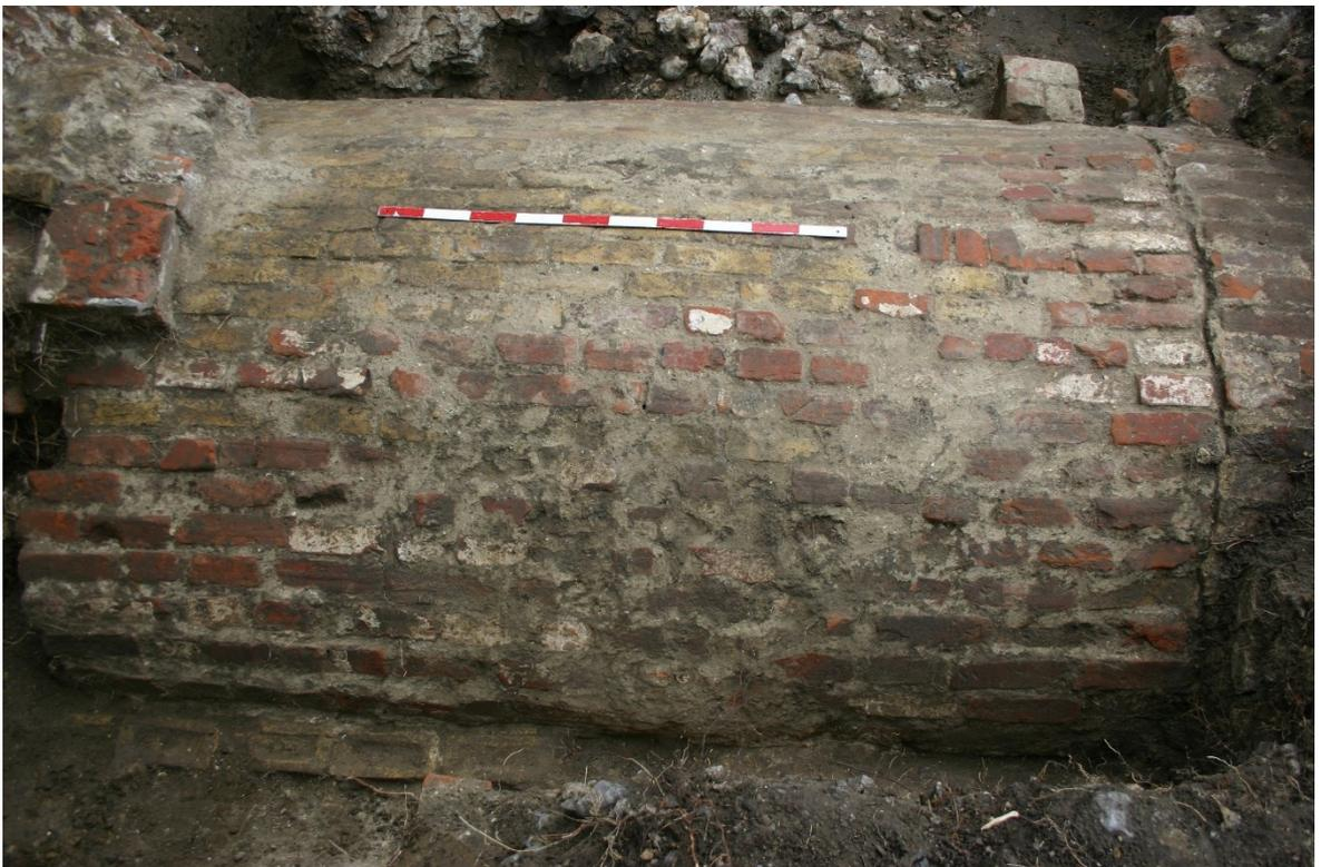
Figure 197. The north side of culvert section 2 before removal. The bonding break with section 1 can be seen on the right.
