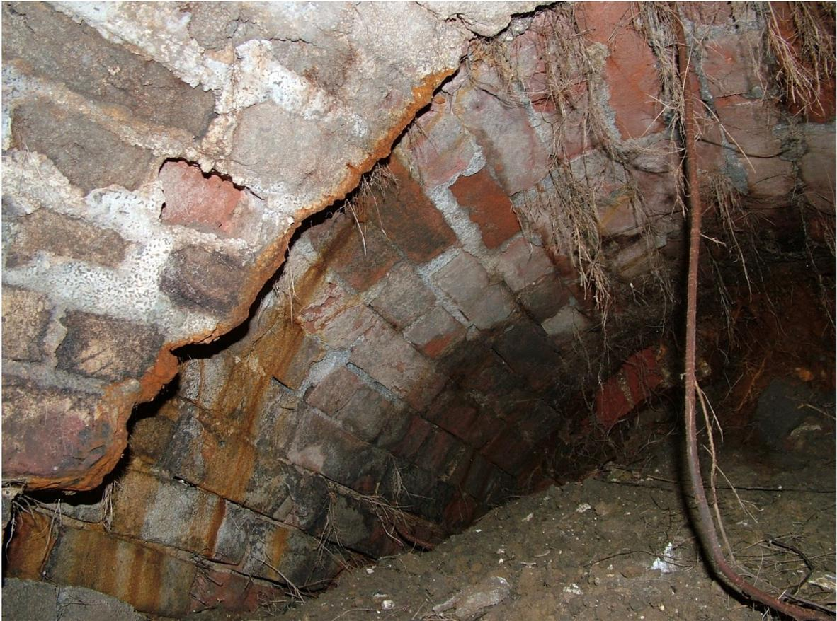
Figure 216. The junction between culvert section 4 and 5 in 2004. Section 4 ended in a fracture. Section 5 turned northwards but soon ended at a collapse.
