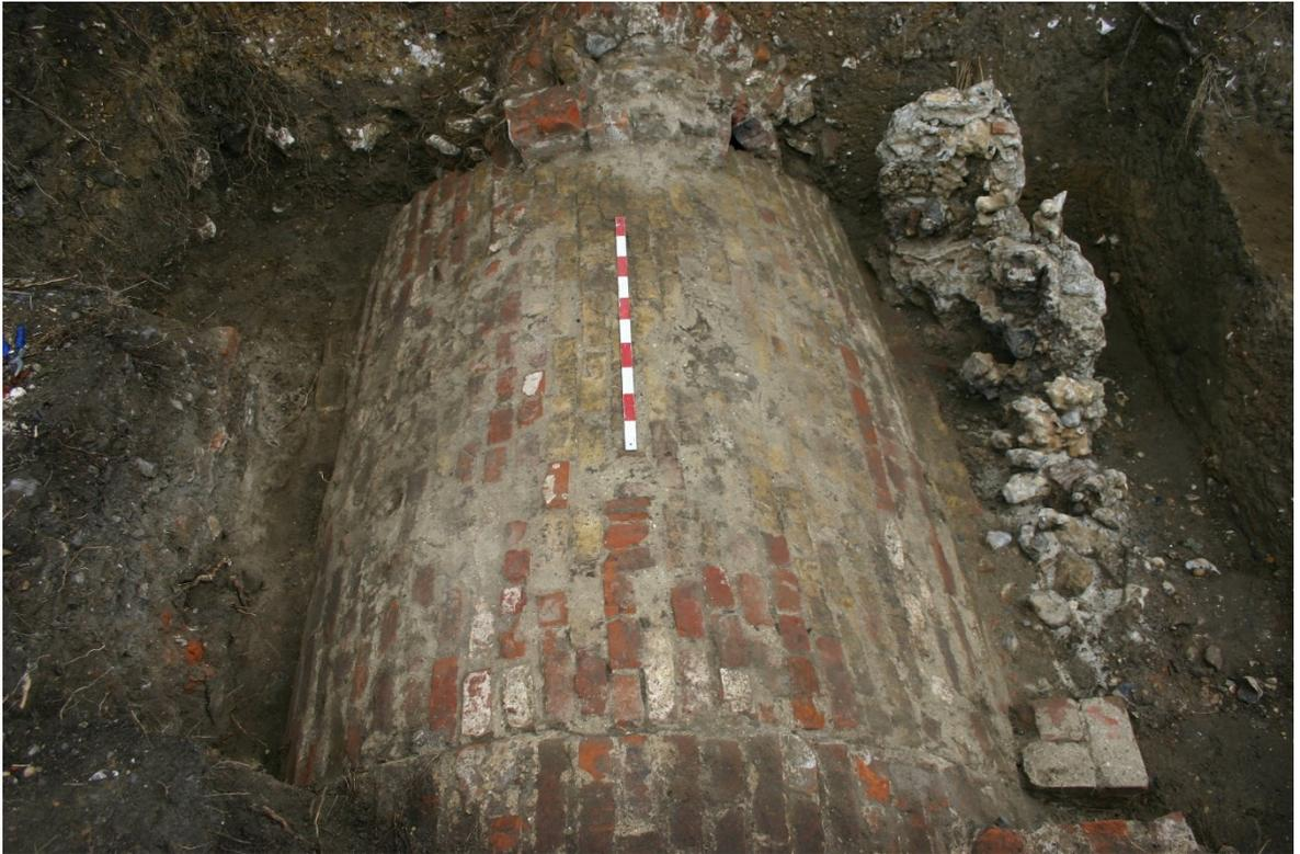
Figure 196. Culvert section 2 before removal. The bonding break forming the junction with culvert section 1 can be seen in the foreground. Looking east.
