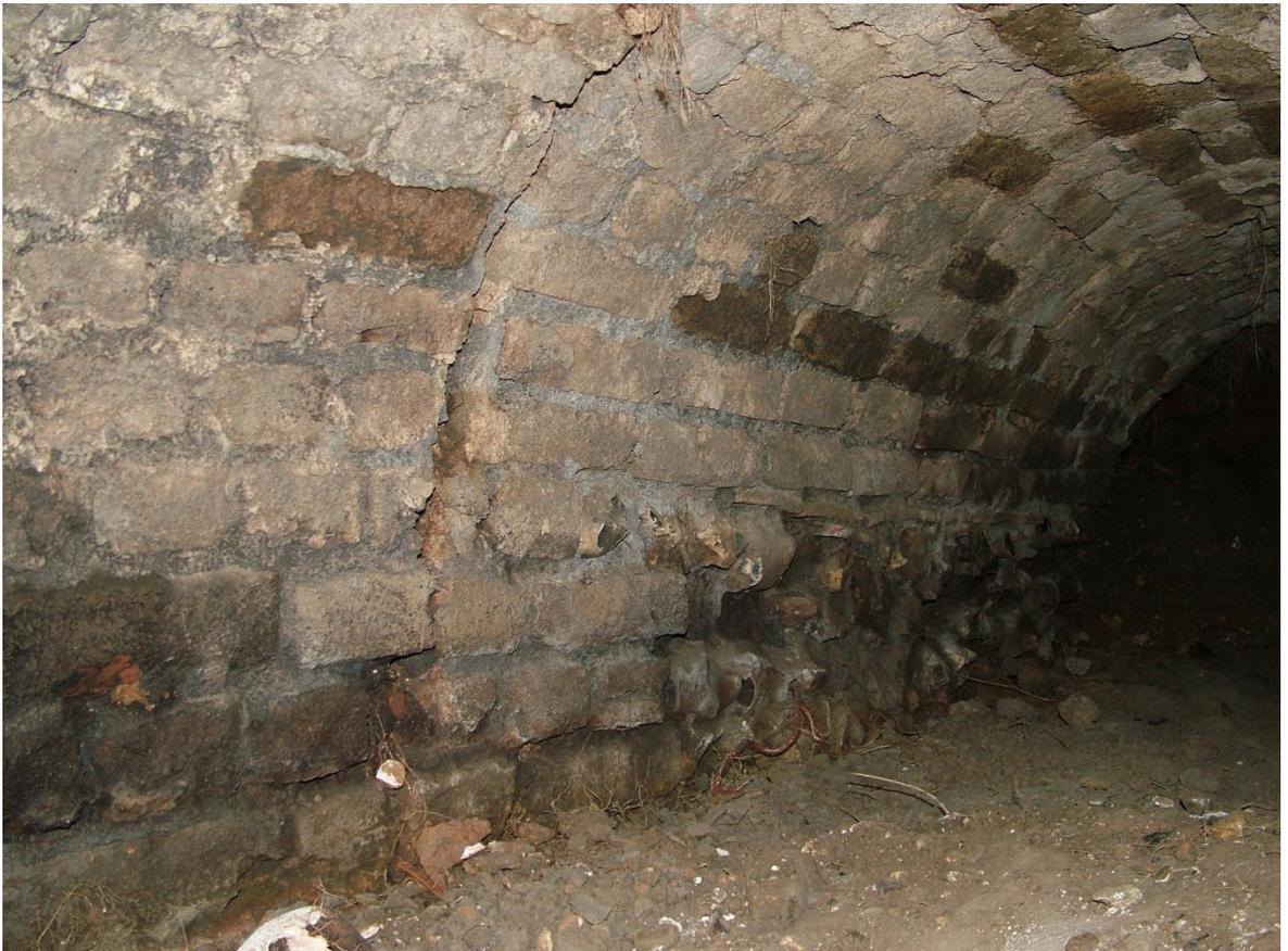
Figure 211. North side of the culvert in 2004, with the crack at the eastern end of section 3, with section 4 to the right.
