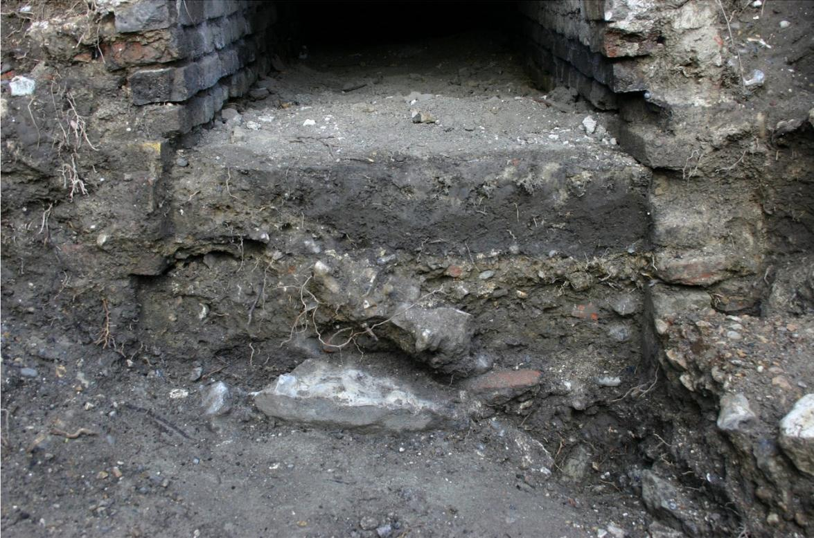
Figure 208. The lower part of the western end of culvert section 3 in 2004, showing how the channel widens below the top of the silt.
