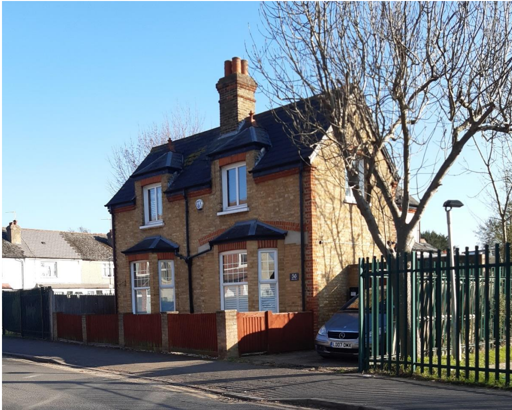
56 Manor Lane as it stands in 2023 (photo by the author)
