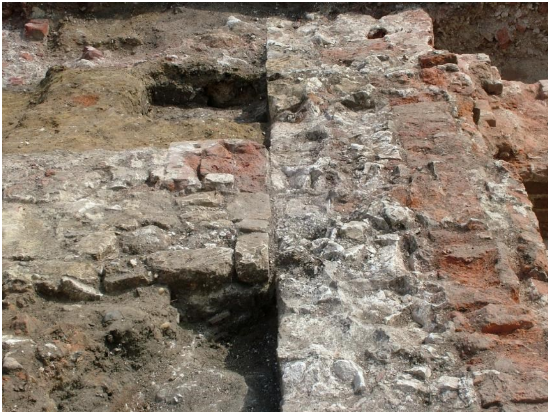
Figure 27. The junction between the north wall of the house (right) and the porch (left).
