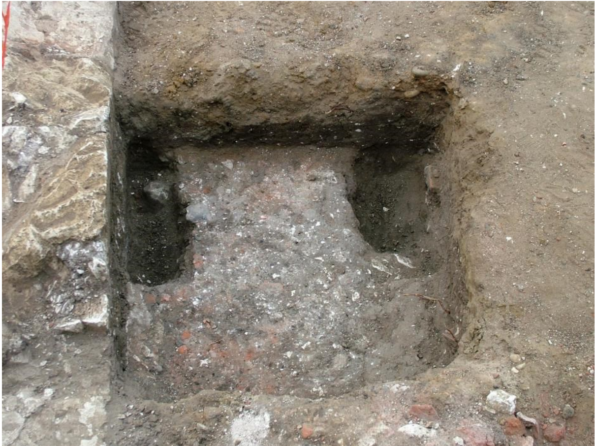
Figure 30. Foundation exposed in the cut excavated in the corner formed by the north wall of the house and the extension built against the north end. The cut appears near the mesh fence on figure 29. Looking west.
