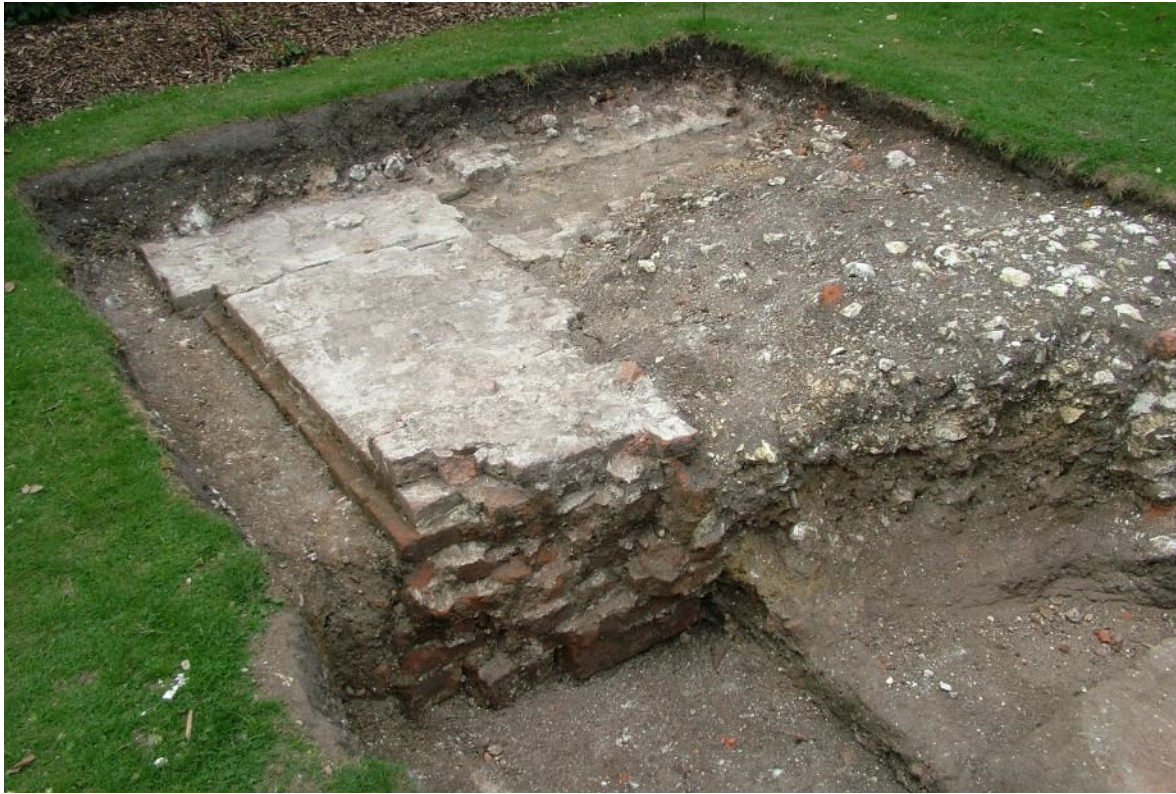
Figure 23. The south end of the trench showing the east wall of the porch. Note the crack in the south end and the two thinner walls at right angles.
