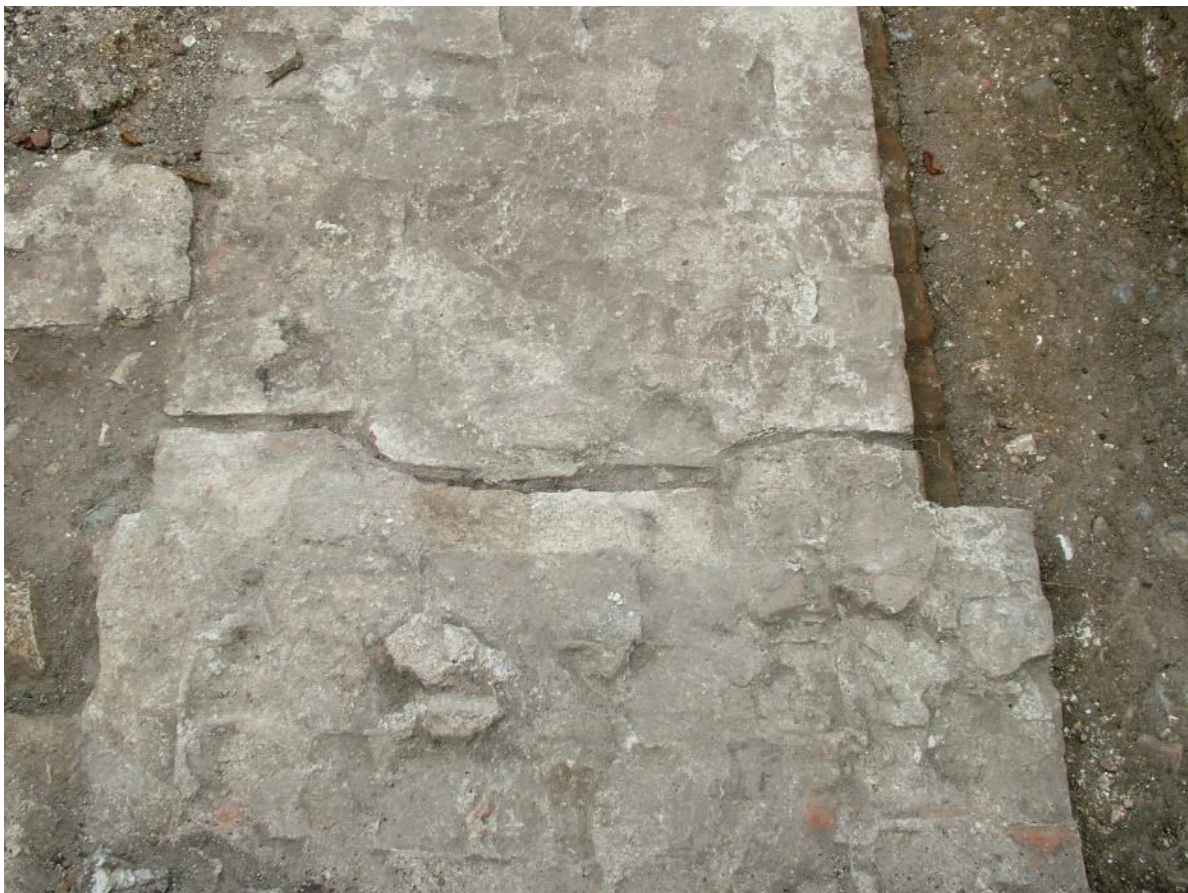
Figure 24. Detail of the crack in the south end of the east wall of the porch. North at the top.
