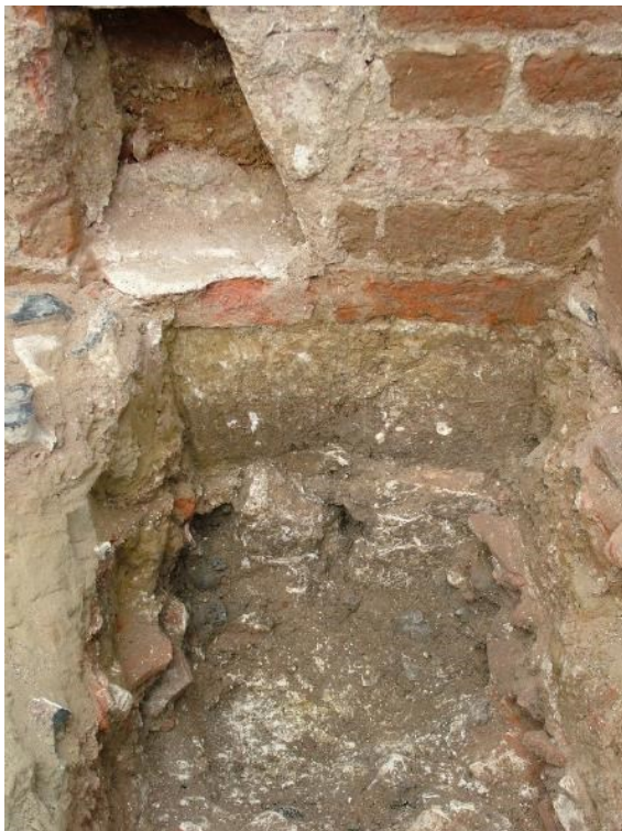
Figure 8. The north side of the sondage in the northeast corner of cellar 1.
