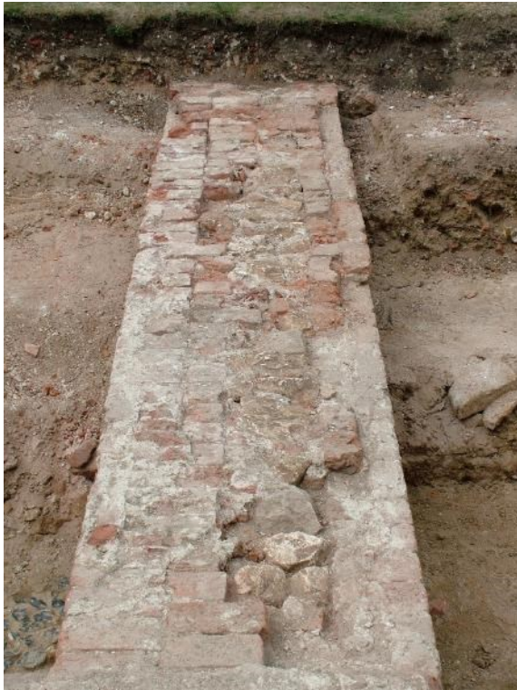
Figure 2. The wall between cellars 1 and 2 looking west.
