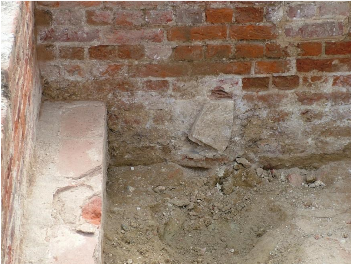
Figure 10. The southeast corner of cellar 1 showing the low wall and the trapezoidal slot with stone (?) set in it.
