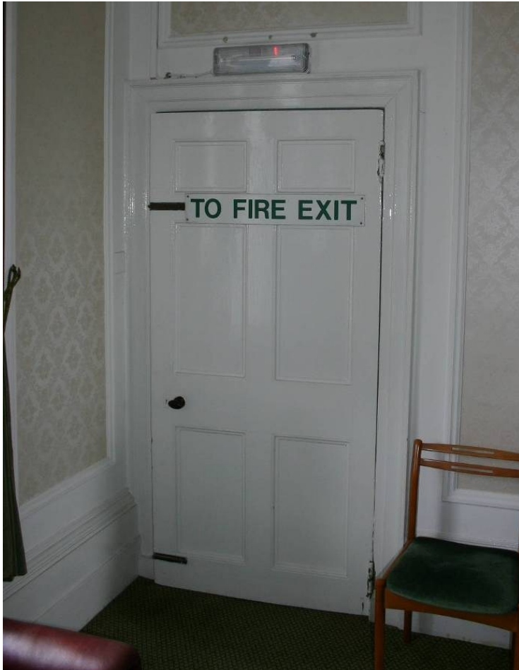
Figure 7. Door between the north wing and the central block.
