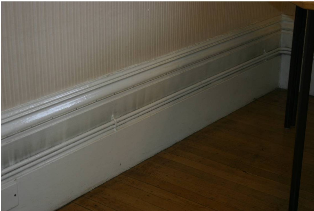
Figure 10. Detail of the skirting on south wall of the south wing.
