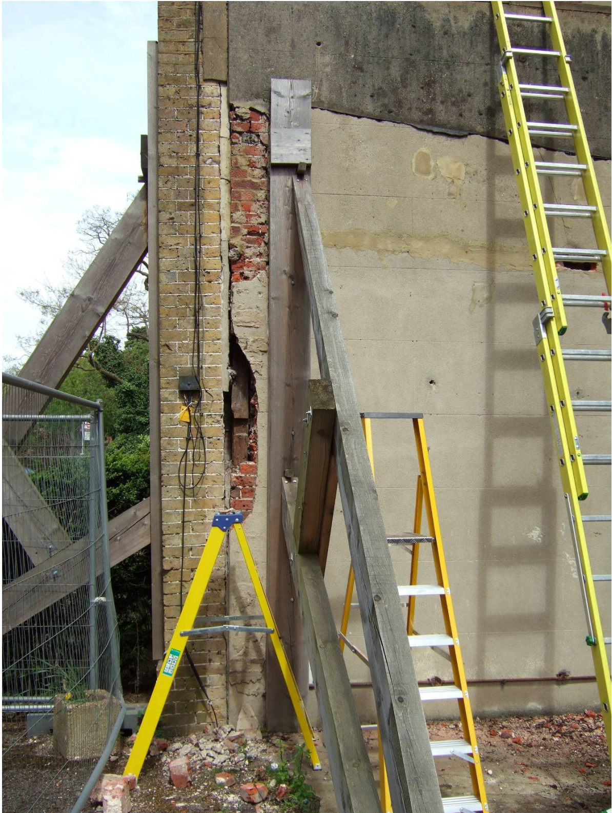
Figure 13. The western end of the south wall of the south wing.
