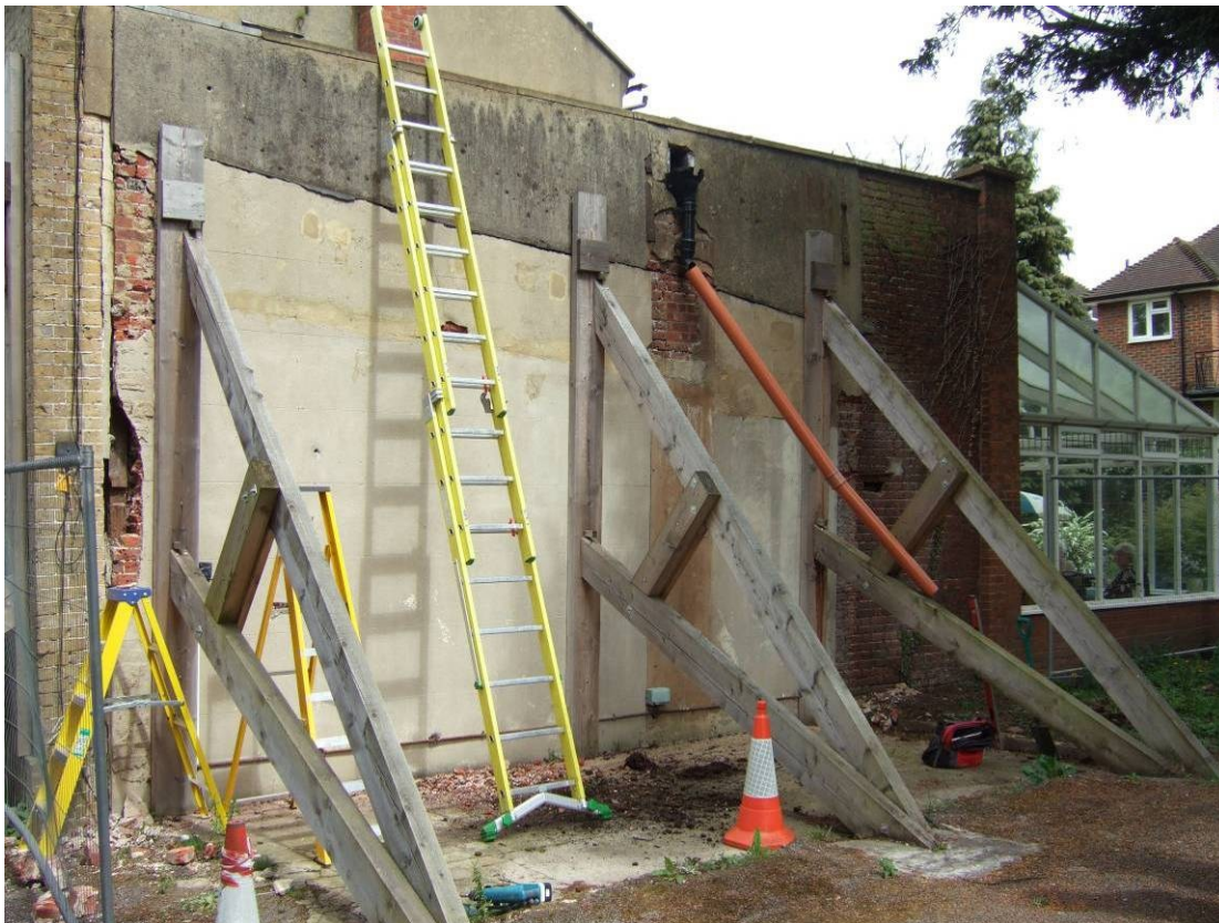
Figure 12. The south wall of the south wing.
