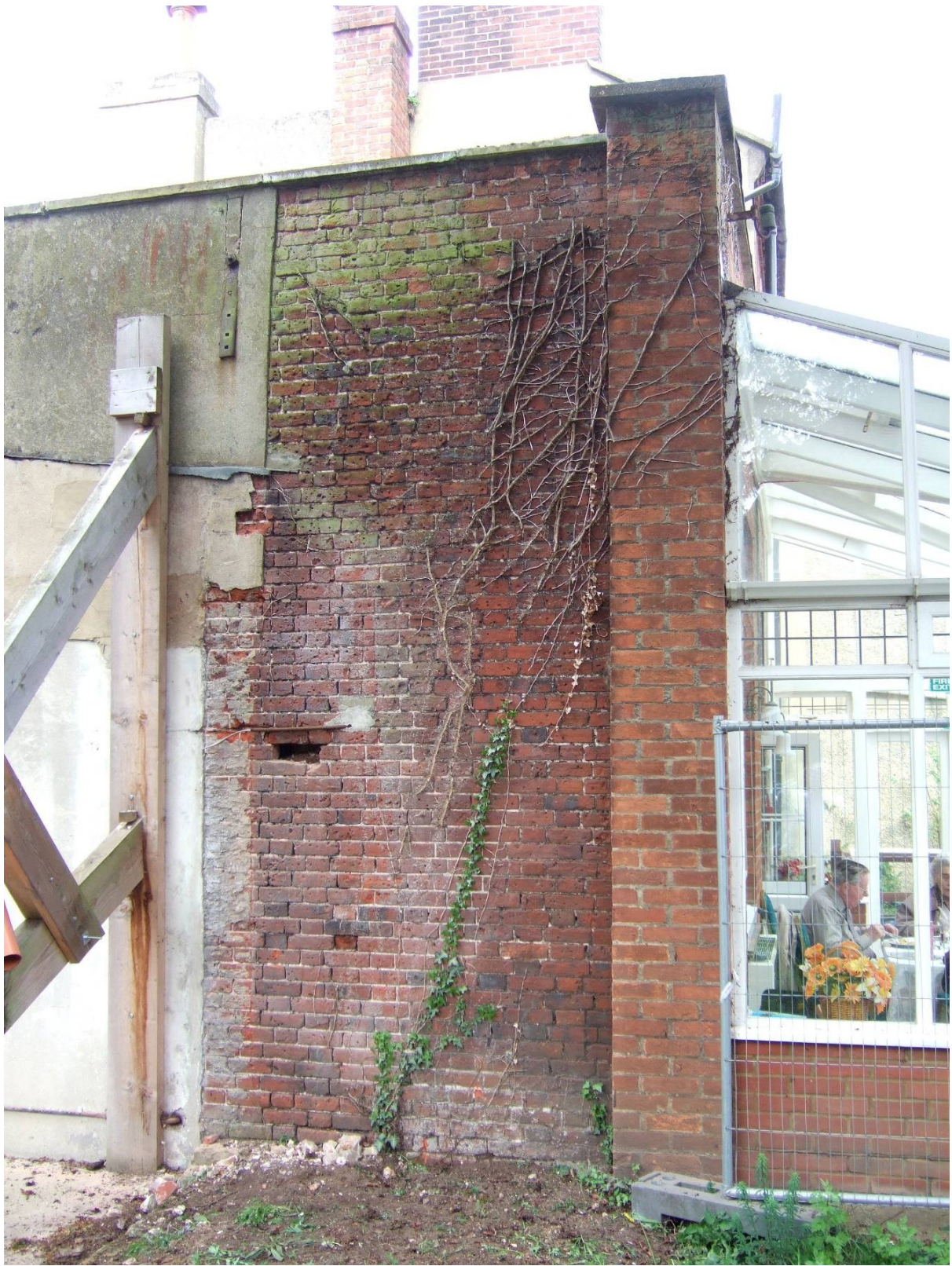
Figure 15. The eastern end of the south wall of the south wing.
